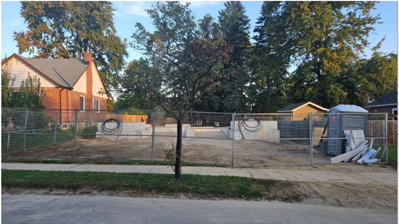
Image 2 – Foundation of Semi-detached dwelling
