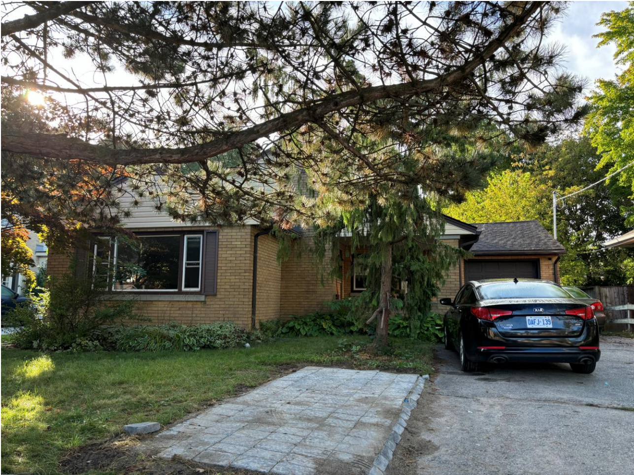
Figure 4: Existing view of 685 Frederick Street from the sidewalk.
