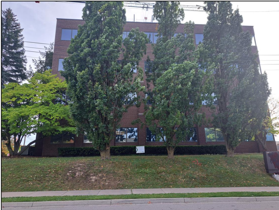
Figure 6: A photo of the side of the building
