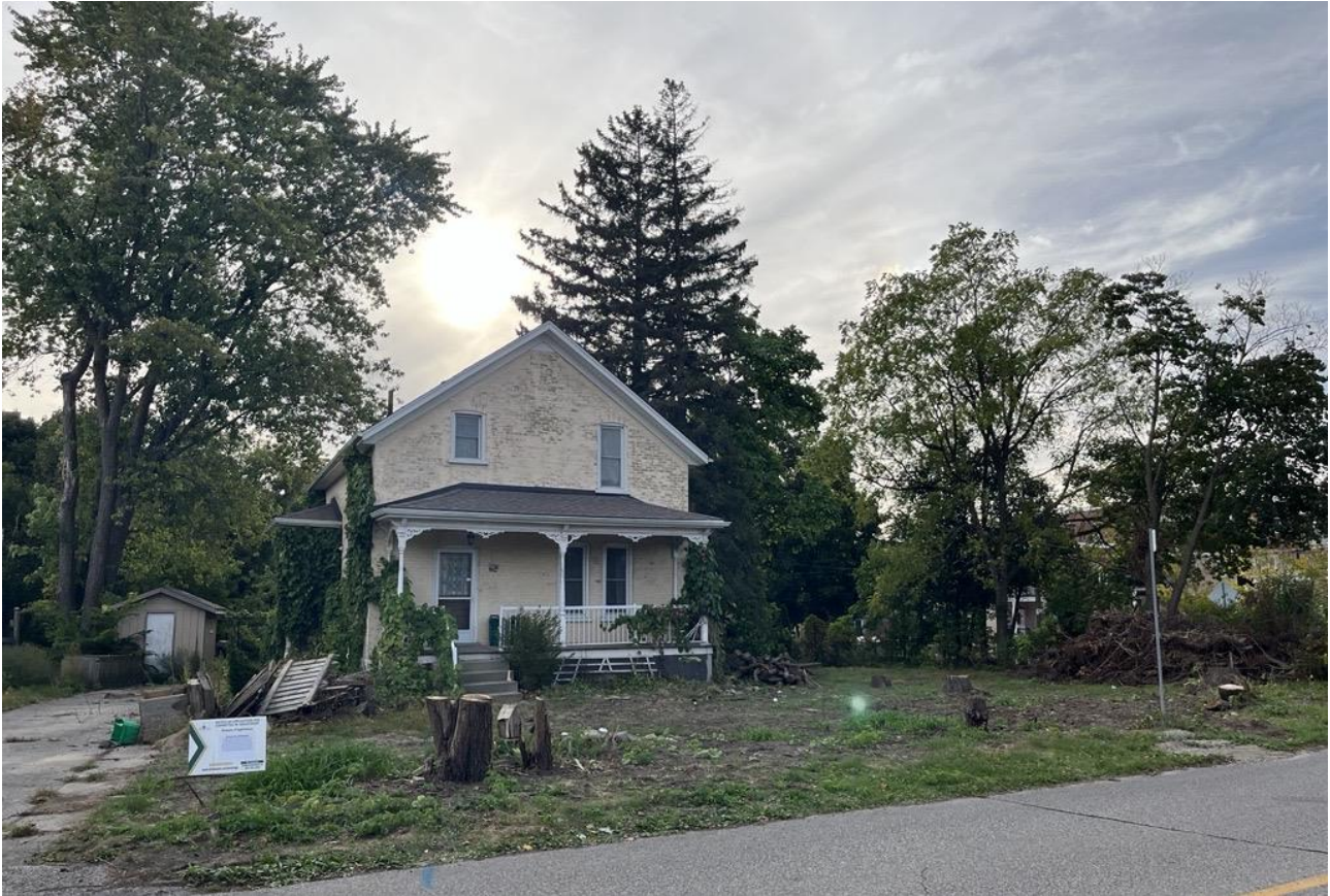
Figure 3: Existing single detached dwelling at 62 Gage Avenue to be demolished
