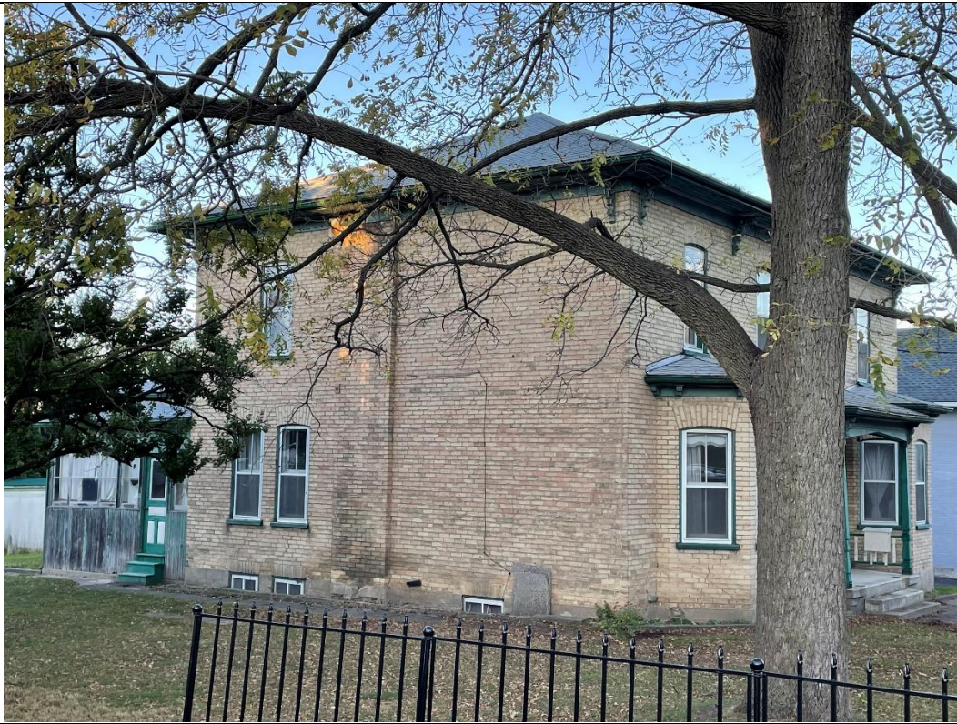
Side Elevation (East Façade) – 79-81 St. George Street
