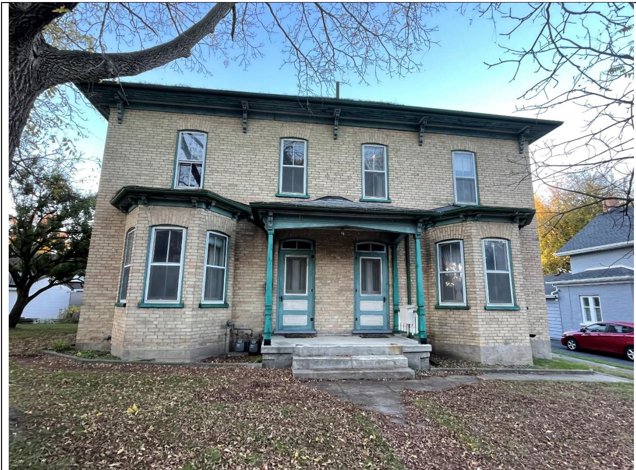
Front Elevation (North Façade) – 79-81 St. George Street
