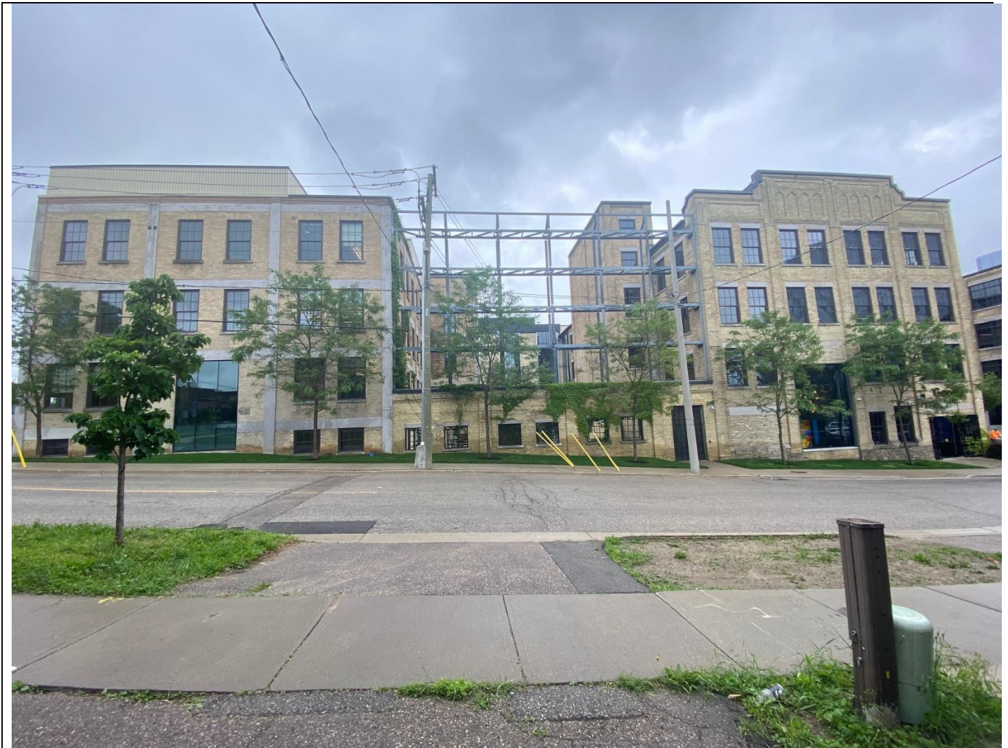
51 Breithaupt Street – front elevation
