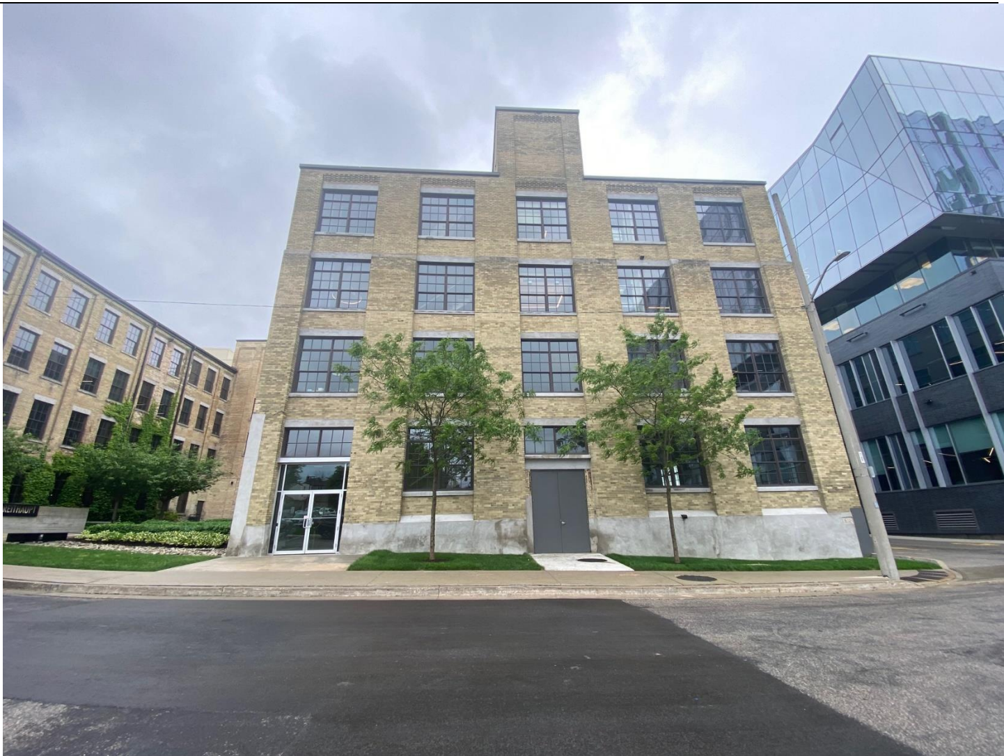
51 Breithaupt Street – front elevation
