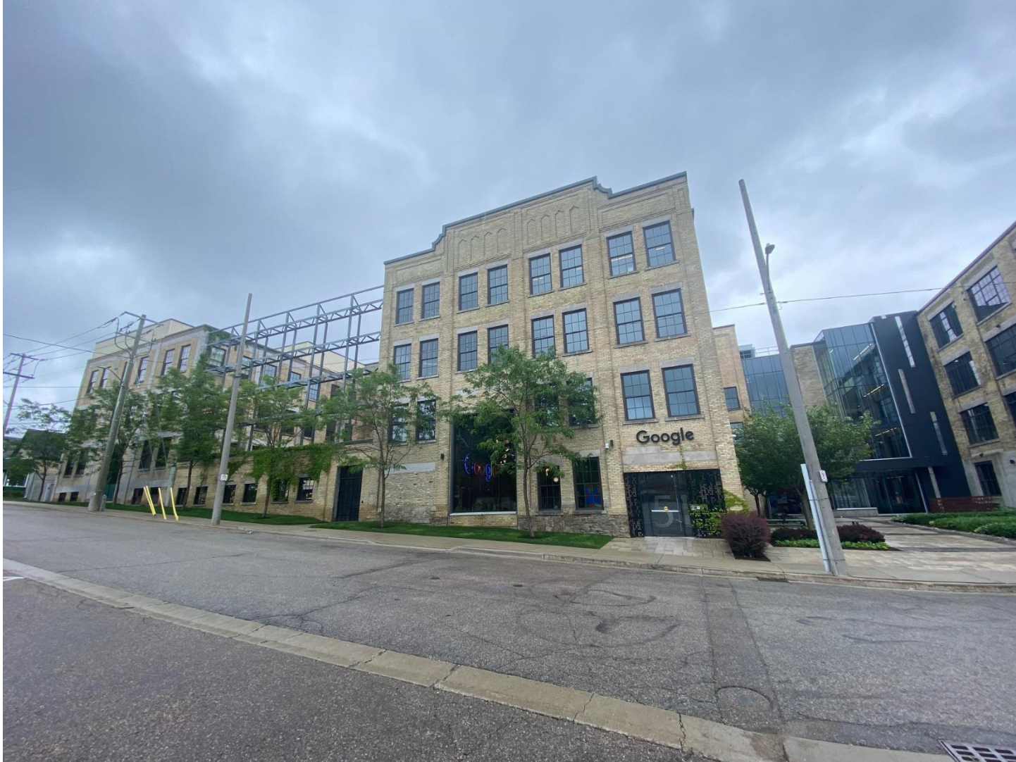
51 Breithaupt Street – front elevation
