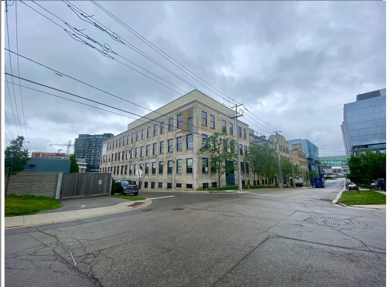
51 Breithaupt Street – front and side elevation
