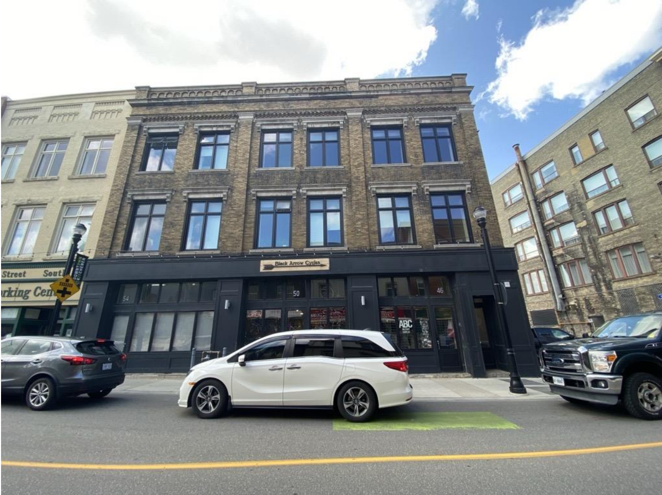
Figure 2. Front Façade of 44-54 Queen Street South
