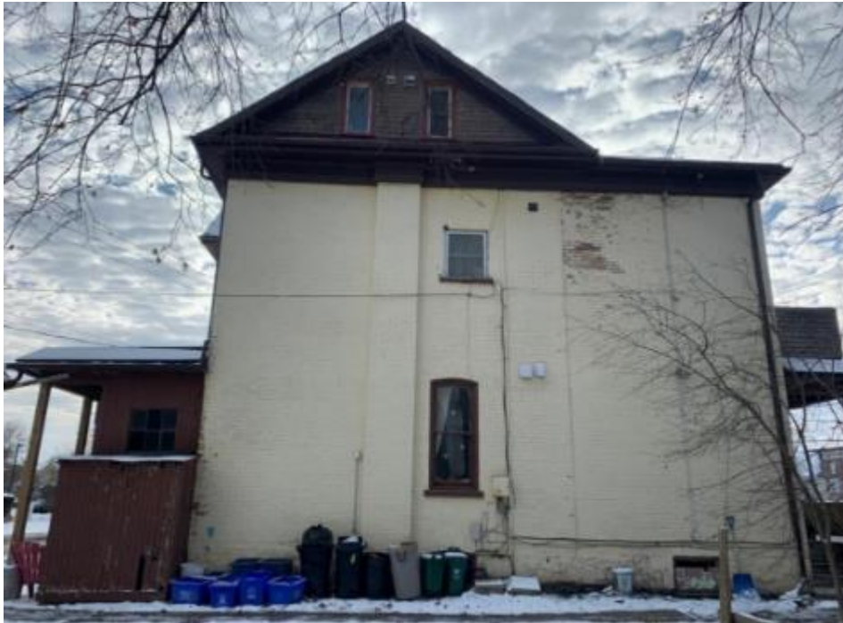
Figure 9. Existing rear (north) facade
