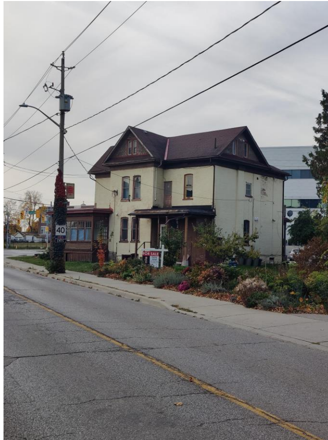
Figure 7. Existing side (east) façade – facing Lancaster Street East
