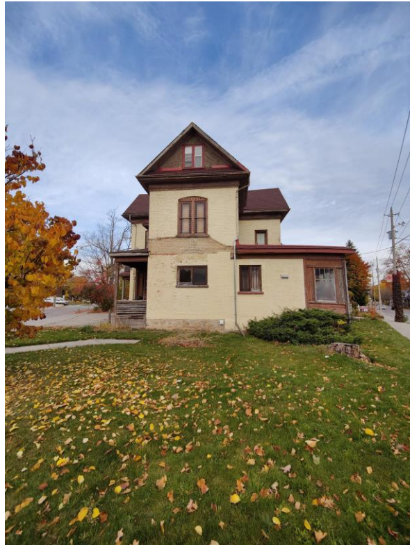
Figure 5. Existing front (south) façade.
