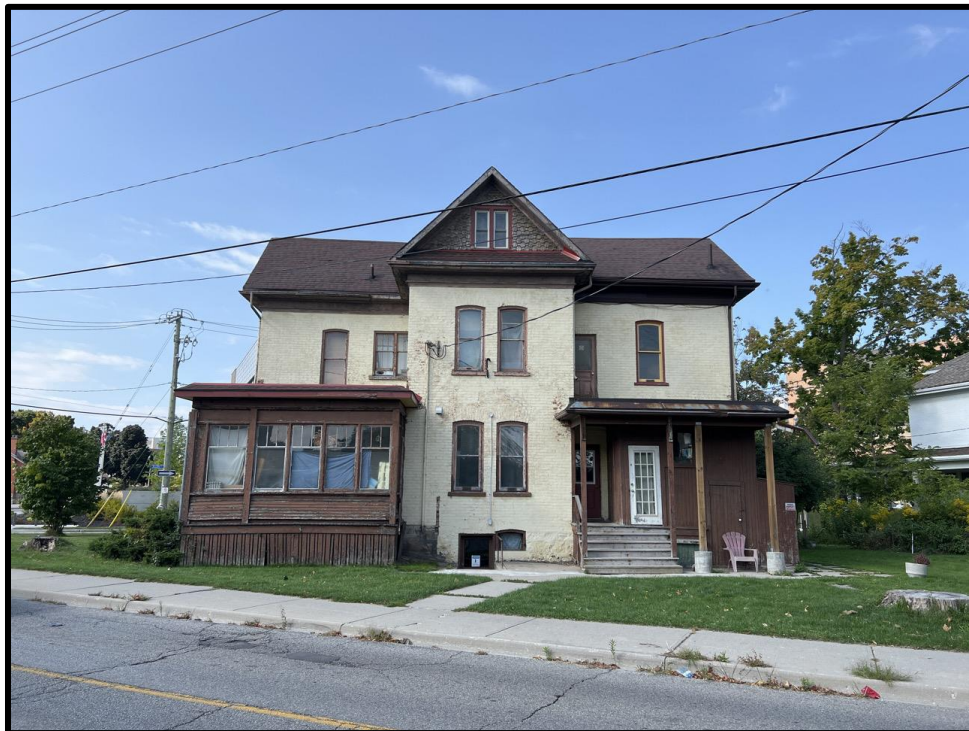
Image 2: Subject Property – East Elevation (Photo taken September 9, 2024)
