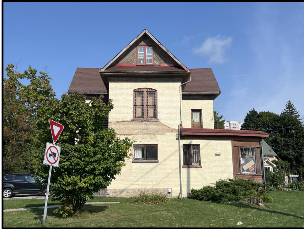
Image 1: Subject Property – Façade (Photo taken September 9, 2024)
