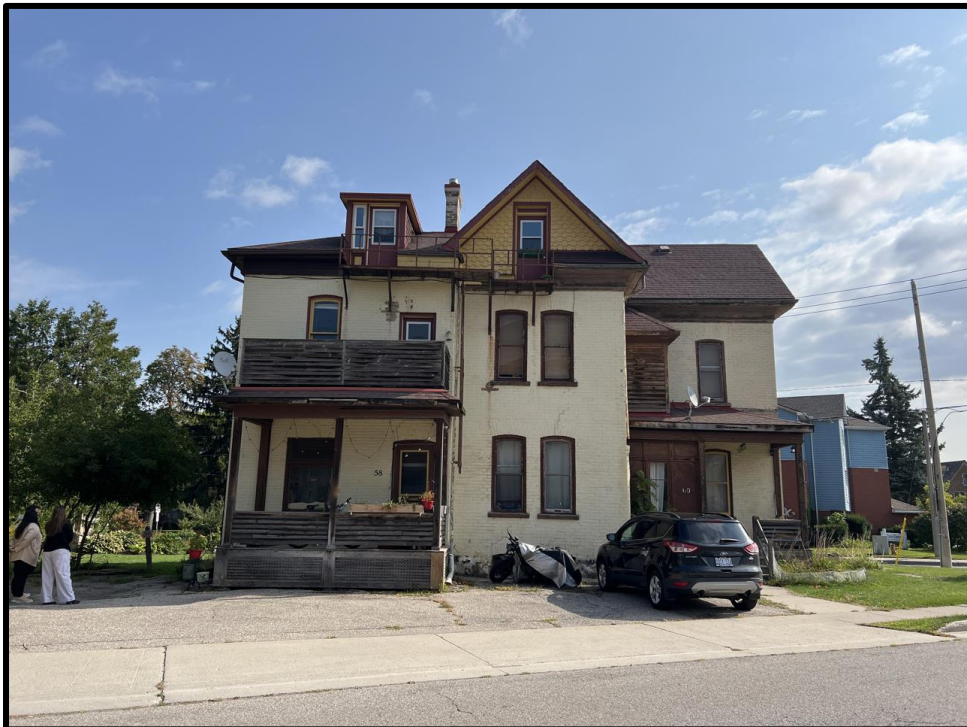
Image 4: Subject Property – West Elevation (Photo taken on September 9, 2024)
