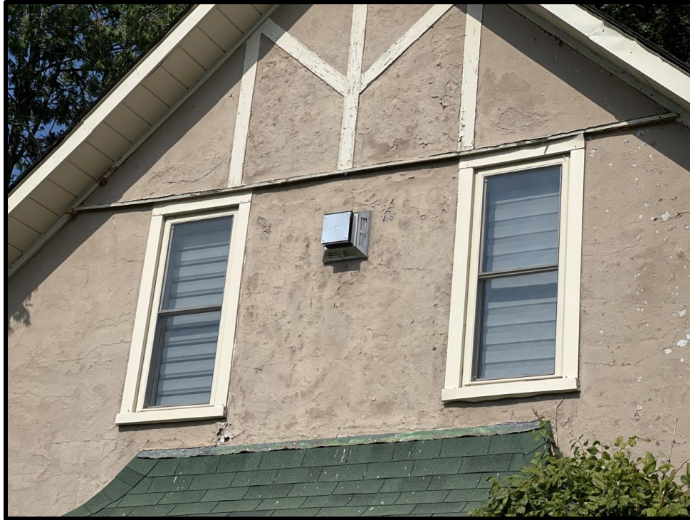
Image 11: Detail of 111 Lancaster Street East (Photo taken September 9, 2024, Facing Northwest)
