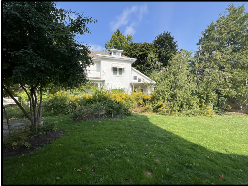
Image 5: 54 Ellen Street East – East Elevation from Subject Property (Photo taken on September 9, 2024, Facing Northwest)
