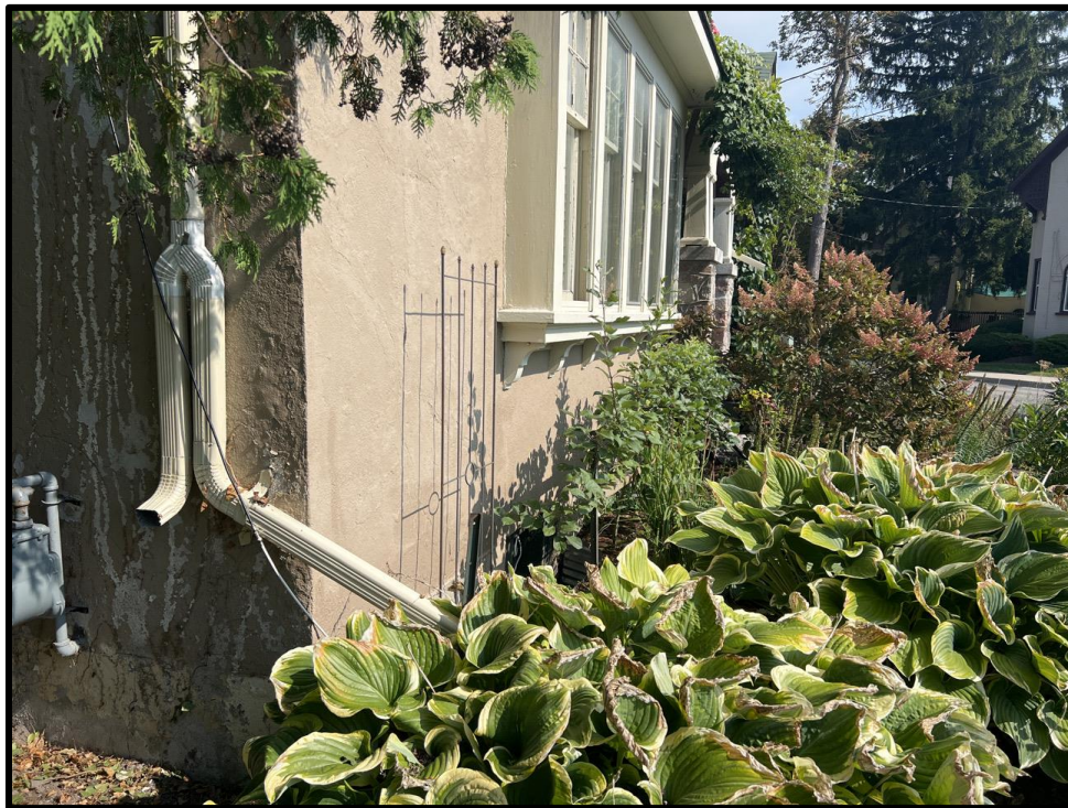
Image 16: Detail of 111 Lancaster Street East from Subject Property (Photo taken September 9, 2024, Facing North)
