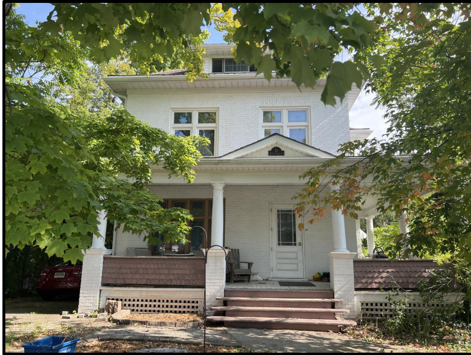
Image 3: 54 Ellen Street East Façade (Photo taken on September 9, 2024, Facing Northeast)
