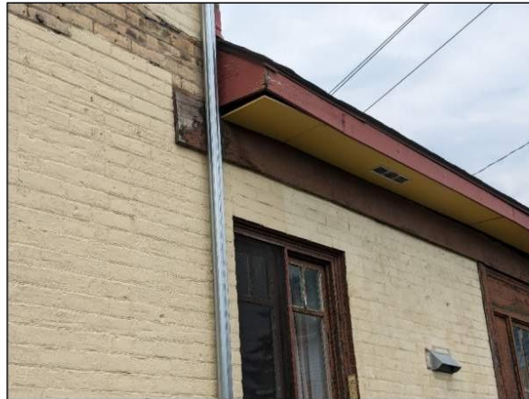
Photograph 4: Loose Soffit
