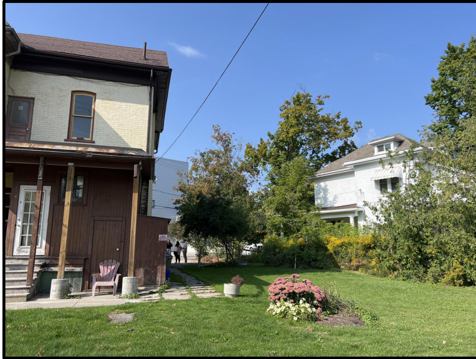
Image 7: View of 54 Ellen Street Through Subject Property from Lancaster Street East (Photo taken September 9, 2024, Facing West)
