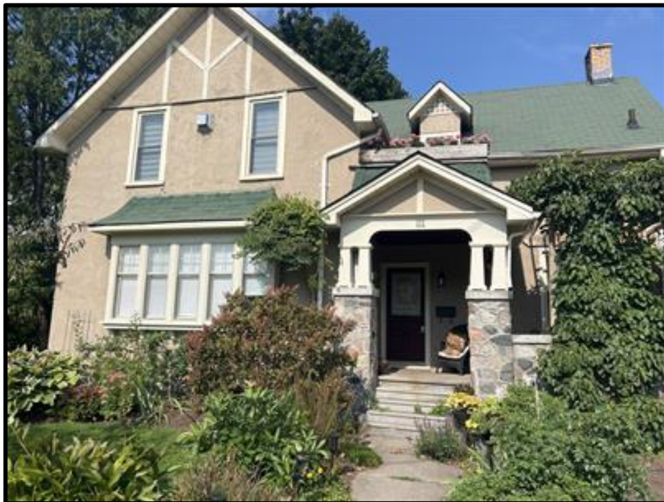
Image 10: 54 Ellen Street East Façade (Photo taken September 9, 2024, Facing Northwest)
