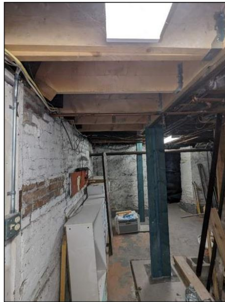
Photograph 16: Typical Basement Conditions
