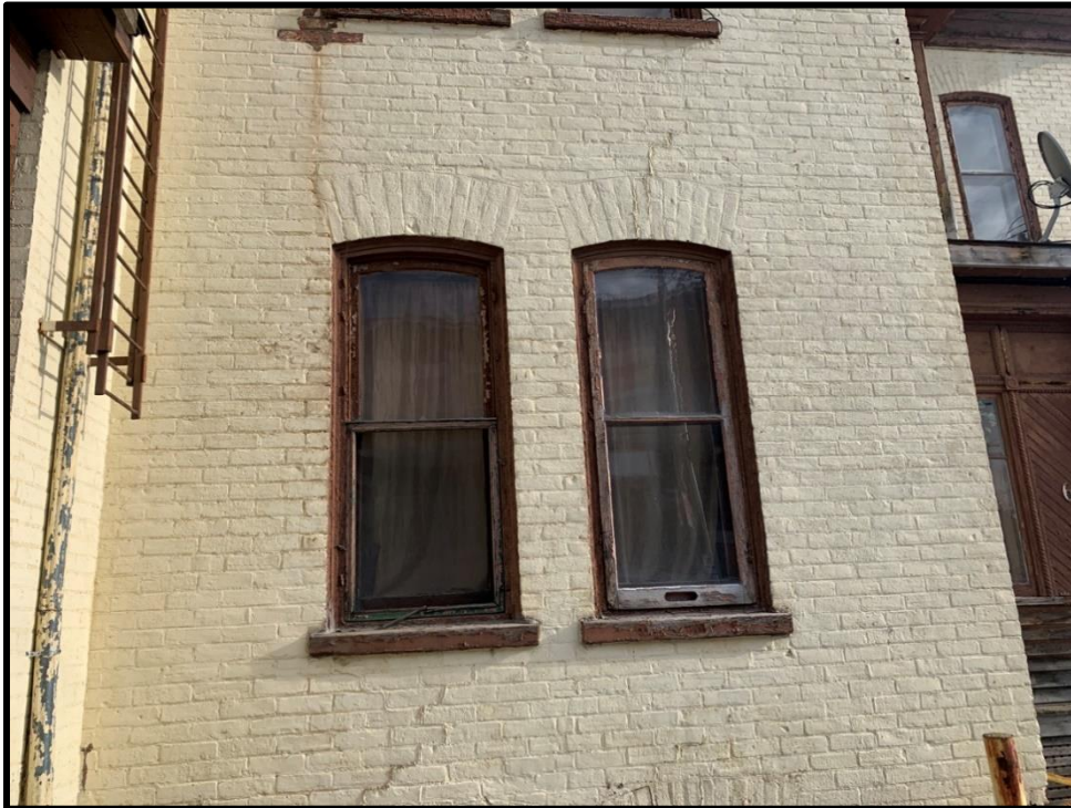
Image 48: Subject Property – Paired Window Openings with Segmental Arches (Photo taken December 20, 2021; Facing East)
