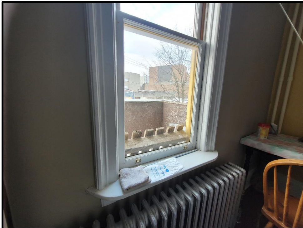
Image 82: 115 Lancaster Street East Interior – Historic Wooden Sash Windows (Photo taken December 20, 2021)
