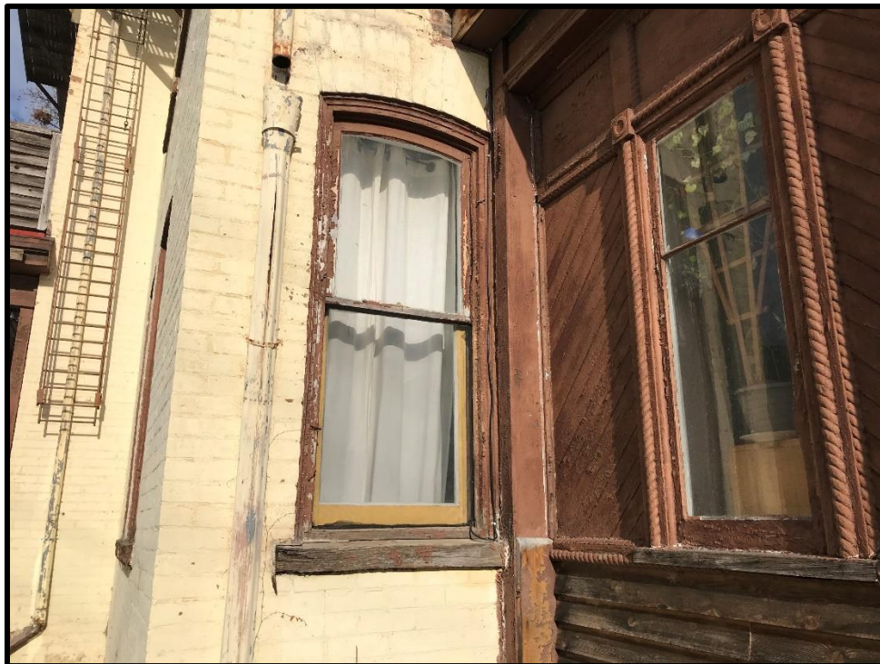
Image 52: Subject Property – One-over-one Wooden Sash Window with Segmental Arch (Photo taken December 20, 2021; Facing North)
