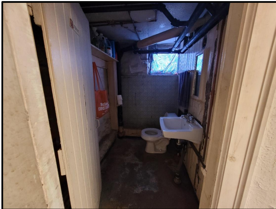
Image 94: Basement – Former Washroom (Photo taken December 20, 2021)
