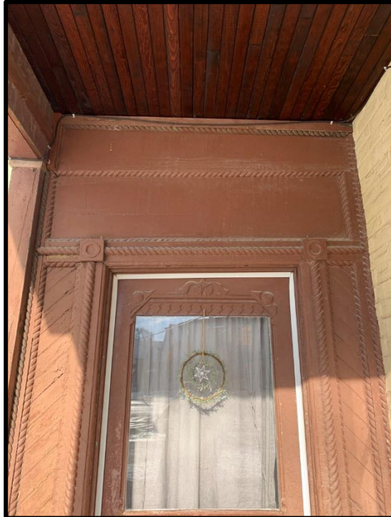
Image 55: Subject Property – 60 Ellen Street Porch with Beadboard Wooden Ceiling (Photo taken December 20, 2021; Facing North)
