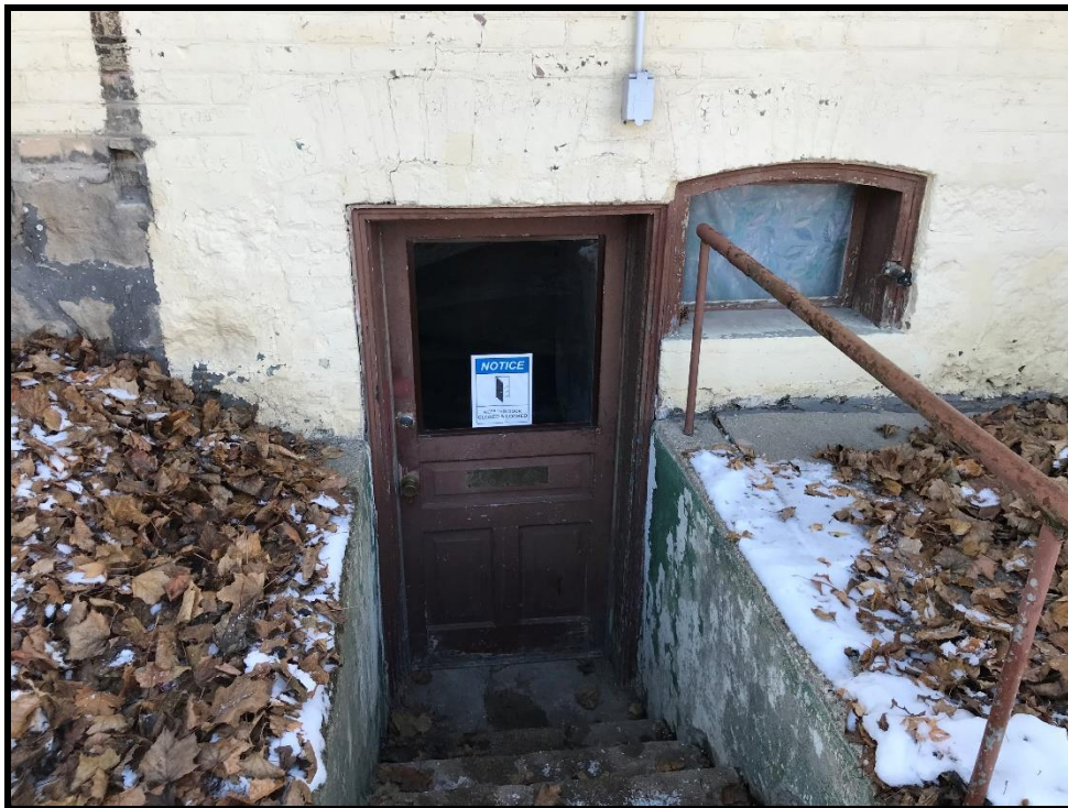
Image 26: Subject Property – Basement Door Showing Modified Opening (Photo taken December 20, 2021; Facing West)
