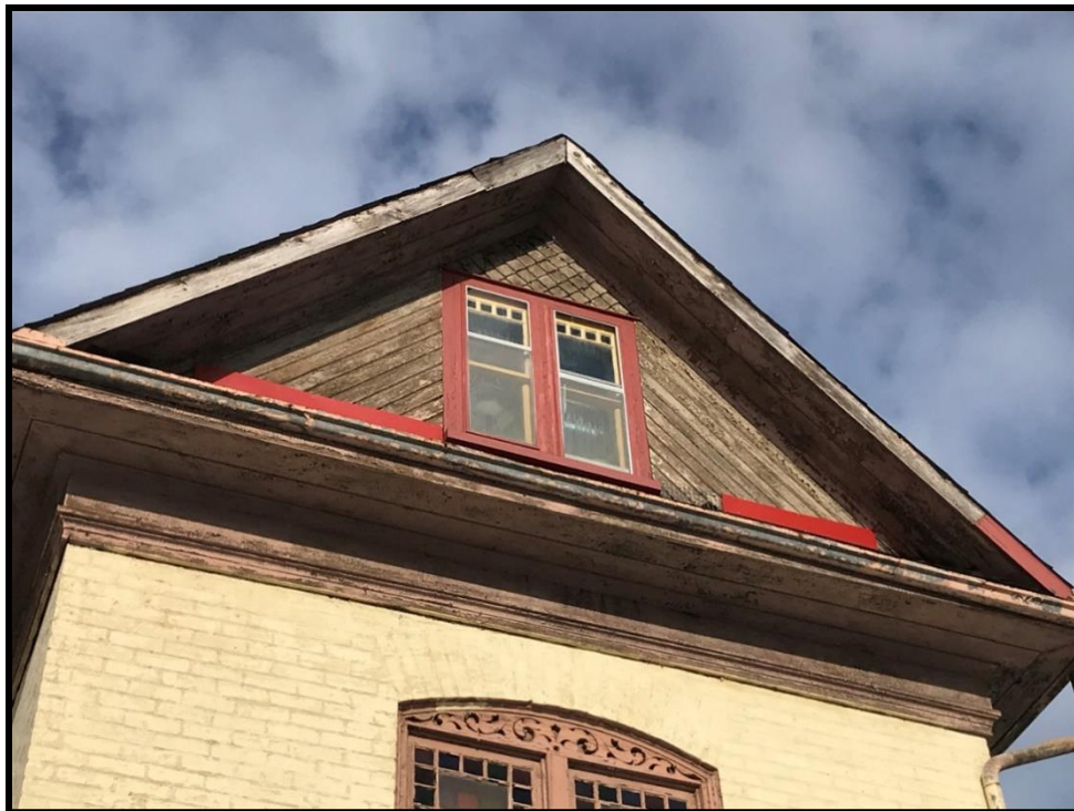
Image 8: Subject Property – Decorative Shingles on Gable End/Multipaned Queen-Anne Style Attic Window (Photo taken December 20, 2021; Facing North)
