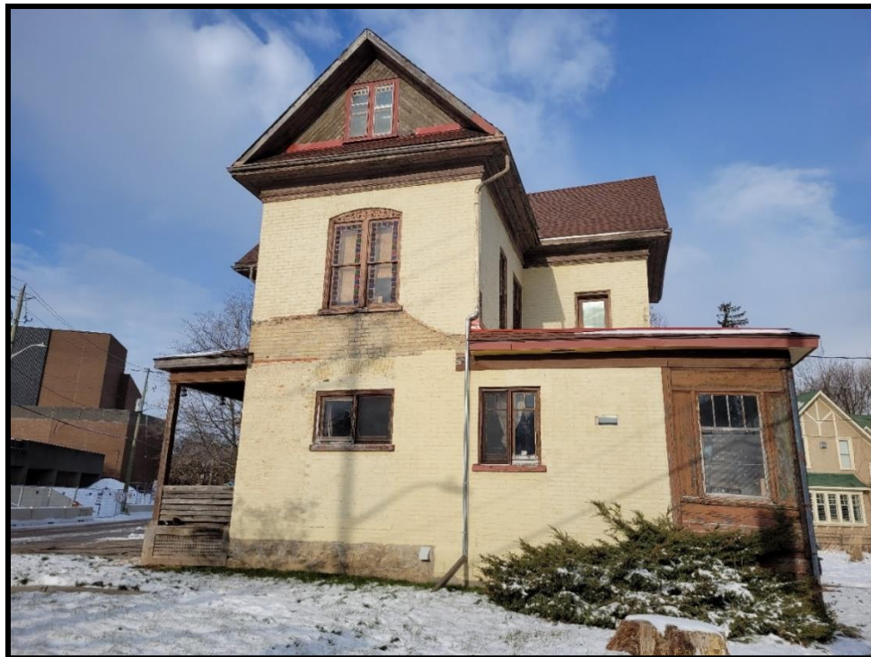
Image 12: Subject Property – Addition on East Corner (Photo taken December 20, 2021; Facing Northwest)
