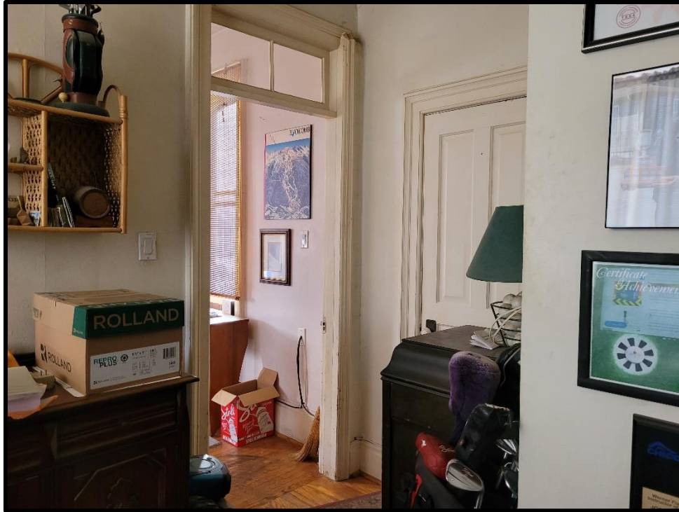
Image 87: 115 Lancaster Street East Interior – Historic Trim and Interior Door Transom, Four-Panel Wooden Door (Photo taken December 20, 2021)
