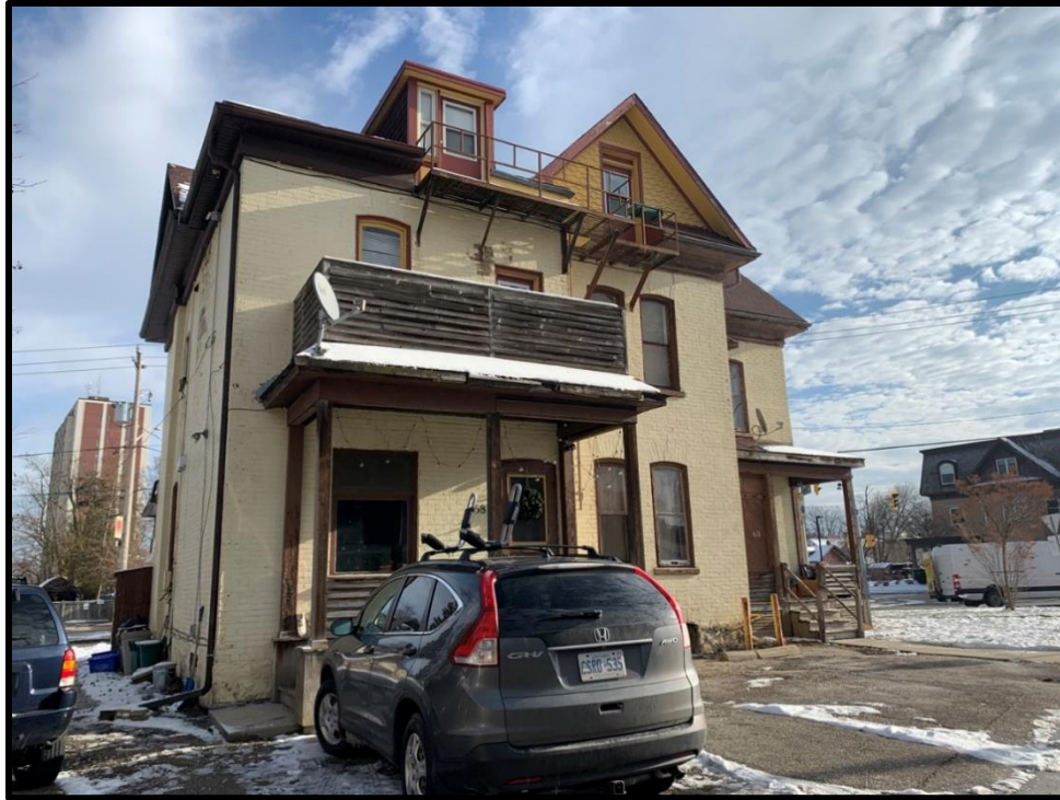
Image 41: Subject Property – Southwest Elevation (Photo taken December 20, 2021; Facing East)
