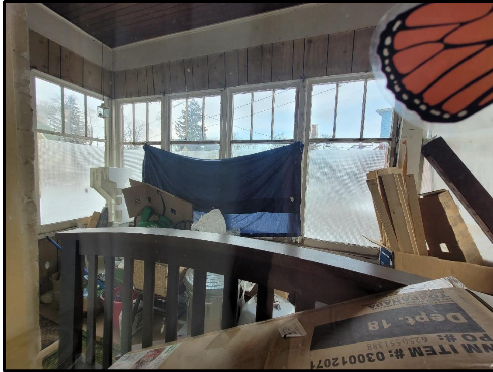
Image 75: 60 Ellen Street East Interior – Addition Interior Area (Photo taken December 20, 2021)
