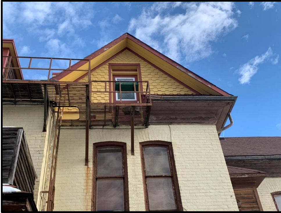
Image 47: Subject Property – Decorative Shingles on Gable End (Photo taken December 20, 2021; Facing East)
