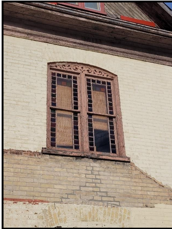
Image 9: Subject Property – Multi-Paned Queen Anne Style Window on Second Storey with Decorative Woodwork (Photo taken December 20, 2021; Facing North)
