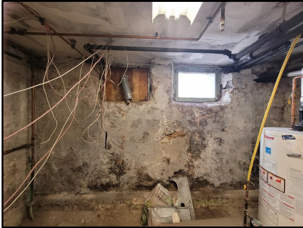
Image 93: Basement – Some Basement Windows Remaining (Photo taken December 20, 2021)
