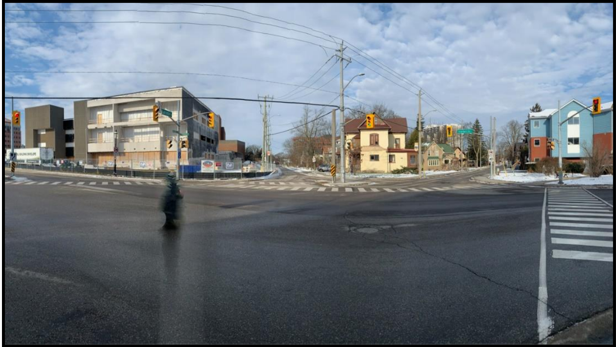
Image 1: Context – View Showing Subject Property from Five Points Intersection (Photo taken December 20, 2021; Facing Northwest)
