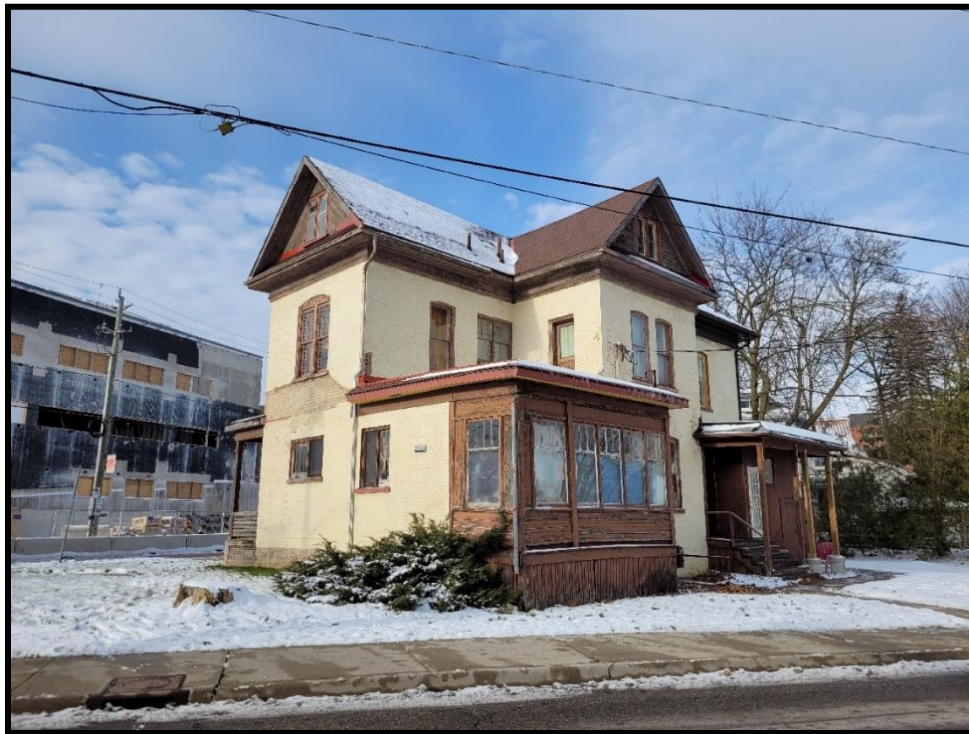
Image 14: Subject Property – East Elevation (Photo taken December 20, 2021; Facing West)
