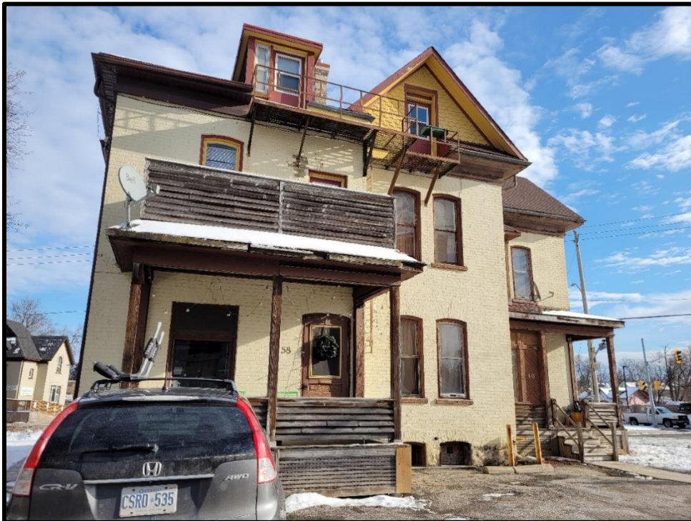
Image 44: Subject Property – First Storey Porch (Photo taken December 20, 2021; Facing East)
