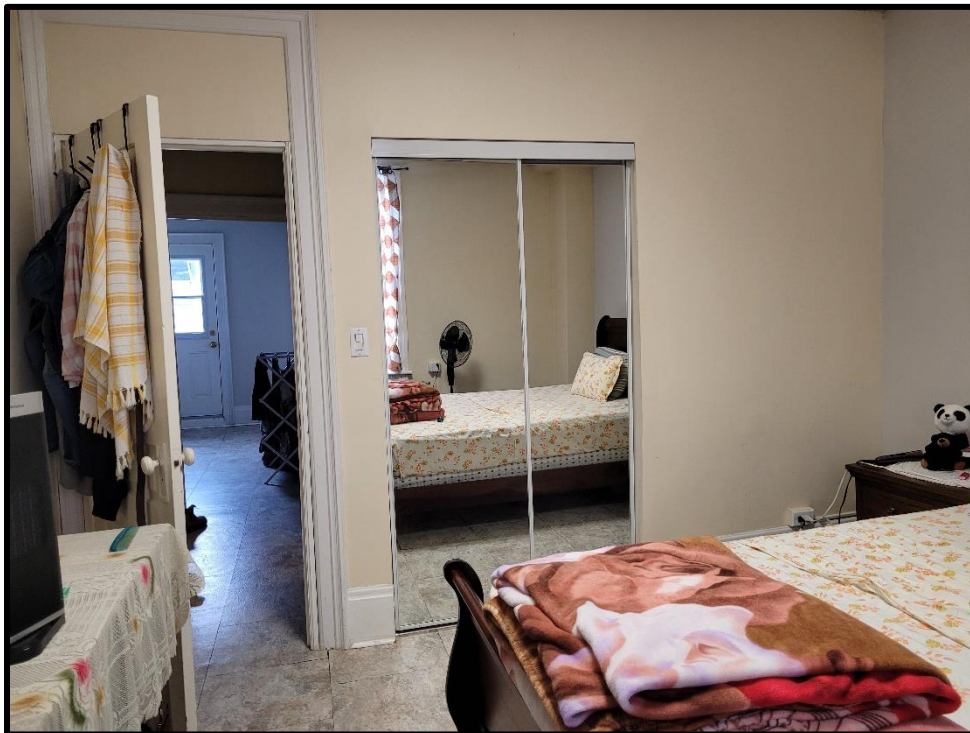
Image 84: 115 Lancaster Street East Interior – Historic Trim and Interior Door Transom (Photo taken December 20, 2021)
