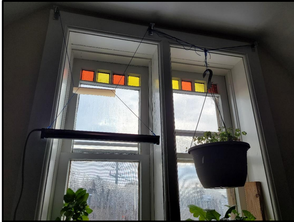
Image 79: 115 Lancaster Street East Interior – Historic Wooden Sash Windows with Coloured Glass Panes (Photo taken December 20, 2021)
