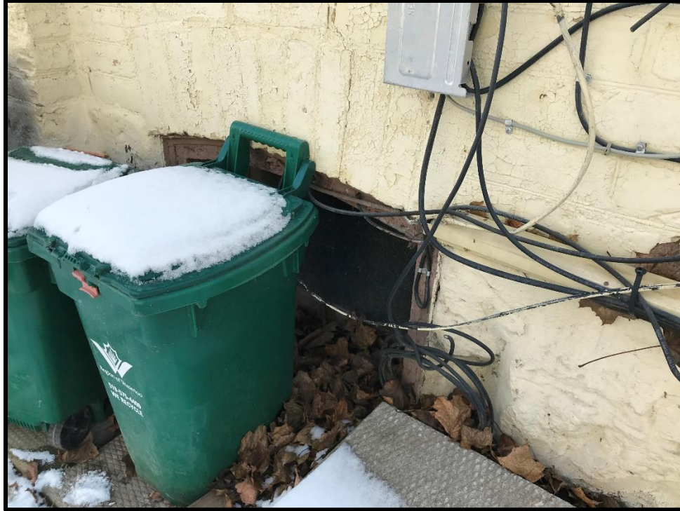
Image 39: Subject Property – Segmental Arch on Basement Opening (Photo taken December 20, 2021; Facing South)
