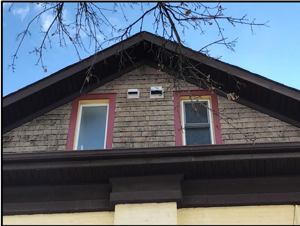
Image 34: Subject Property – Decorative Shingles on Gable Ends (Photo taken December 20, 2021; Facing Southeast)
