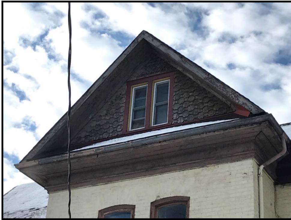
Image 19: Subject Property – Decorative Shingle Work on Gable End (Photo taken December 20, 2021; Facing Southwest)
