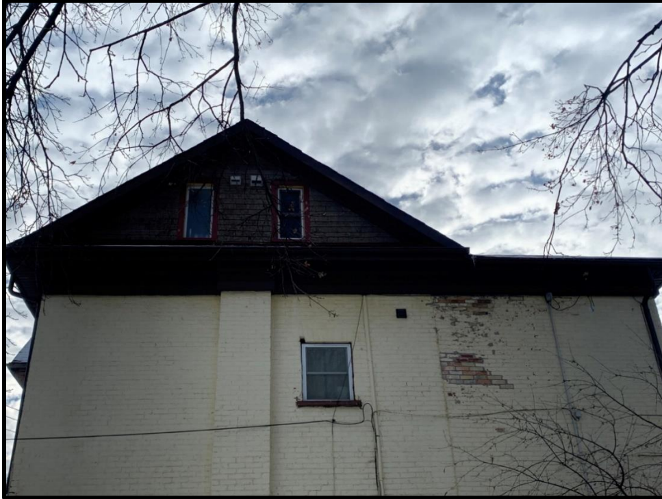
Image 33: Subject Property – Outside Brick Chimney (Photo taken December 20, 2021; Facing Southeast)
