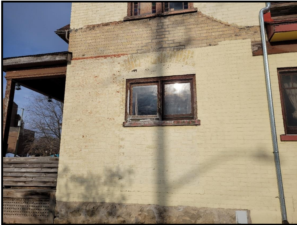
Image 11: Subject Property – Infilled Window Opening (Photo taken December 20, 2021; Facing Northwest)
