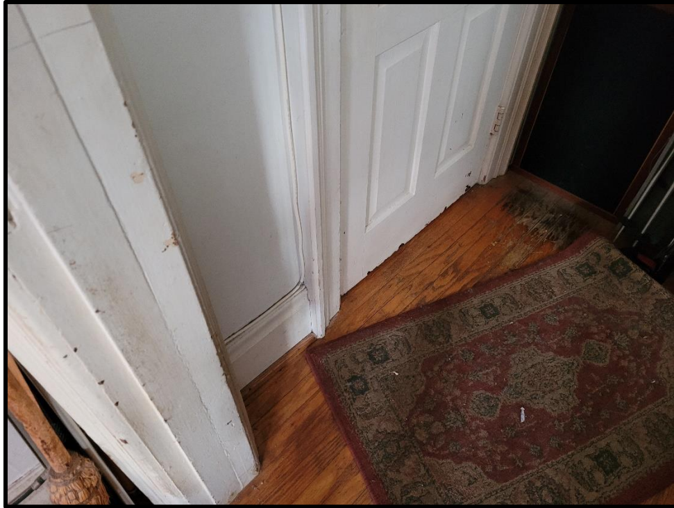
Image 89: 115 Lancaster Street East Interior – Historic Hardwood Flooring (Photo taken December 20, 2021)
