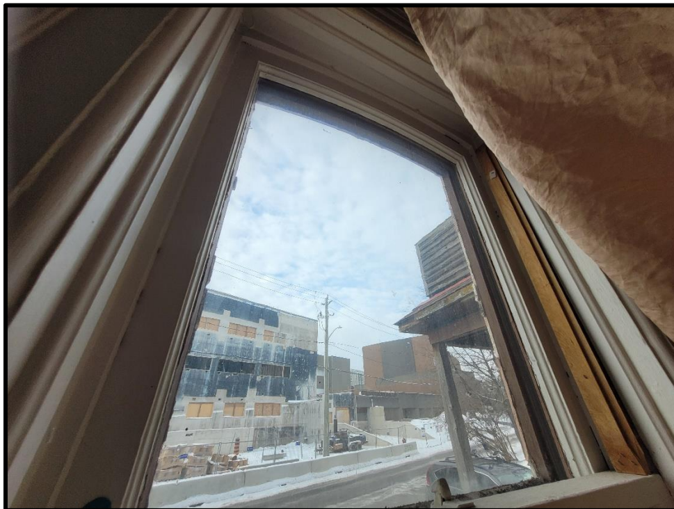
Image 68: 60 Ellen Street East Interior – Wooden Sash Windows with Trim (Photo taken December 20, 2021)
