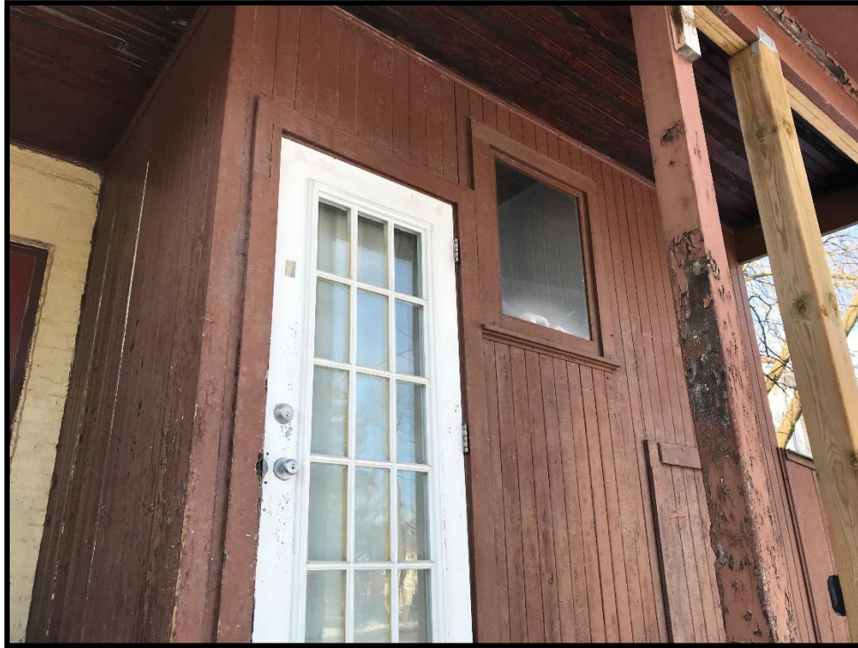
Image 27: Subject Property – Addition on North Corner (Photo taken December 20, 2021; Facing Northwest)
