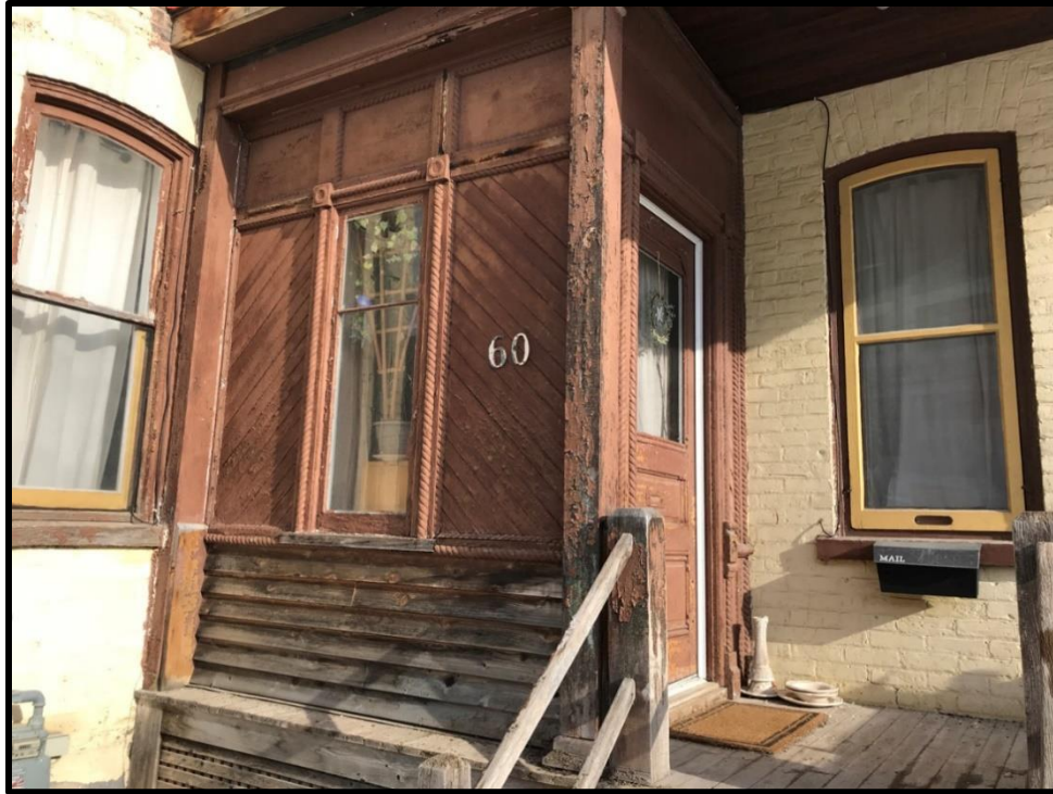
Image 51: Subject Property – 60 Ellen Street Enclosed Entrance (Photo taken December 20, 2021; Facing Northeast)
