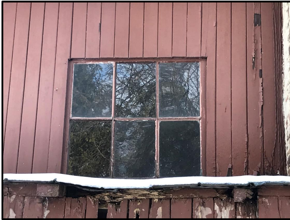
Image 31: Subject Property – Six-Paned Fixed Window on Northwest Elevation of One-Storey Addition (Photo taken December 20, 2021; Facing South)
