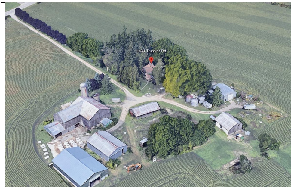
Complex of Farm Buildings Looking North West – 1434 Trussler Road (Source: Google Earth, 2024)
