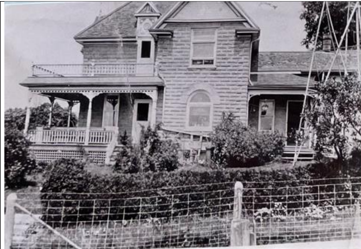
Historic Front Elevation (South Façade) – 1434 Trussler Road (Source: Helena Feasby Women's Institute, 1981)
