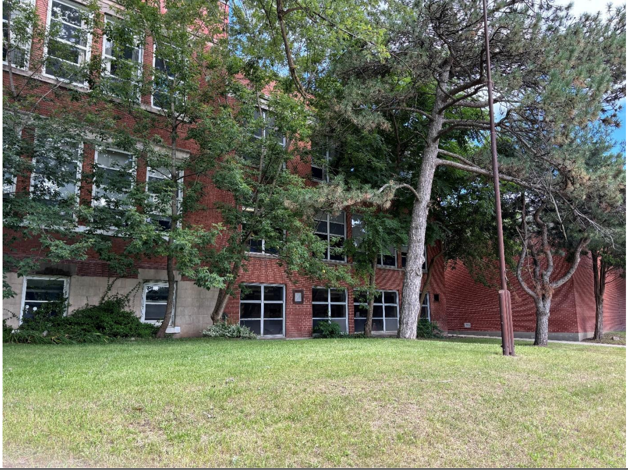
Front Elevation (South) – View of unknown and 1974 addition.
