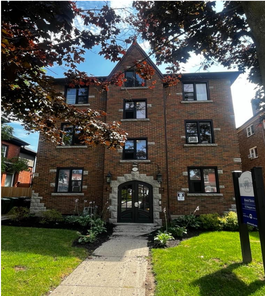
Figure 2: Front Facade of Subject Property
