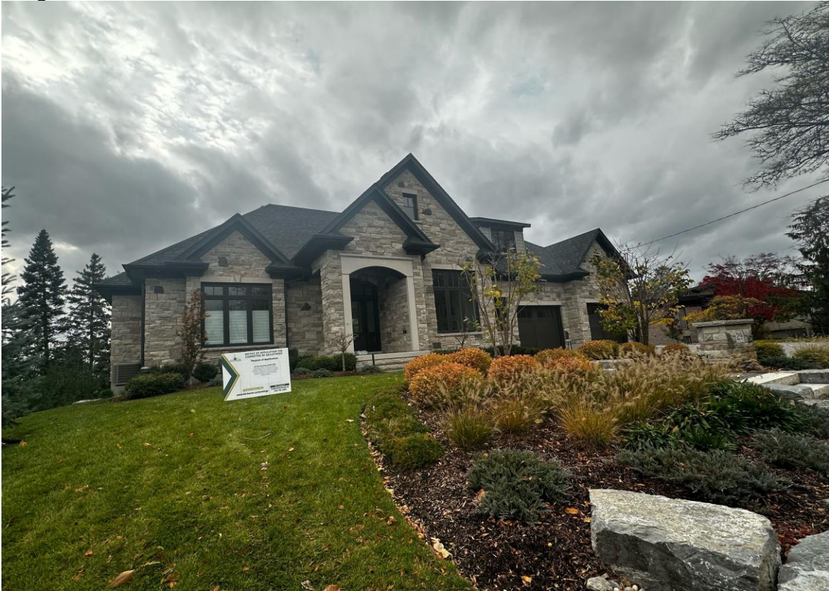
Figure 4: Existing Site Conditions at 29 The Crestway on October 31, 2024
