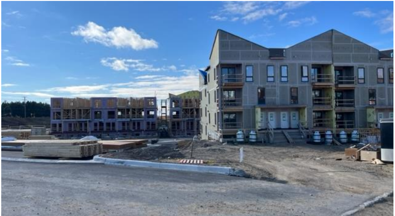
Figure 5: Future townhouses under construction – 630 Benninger Drive
