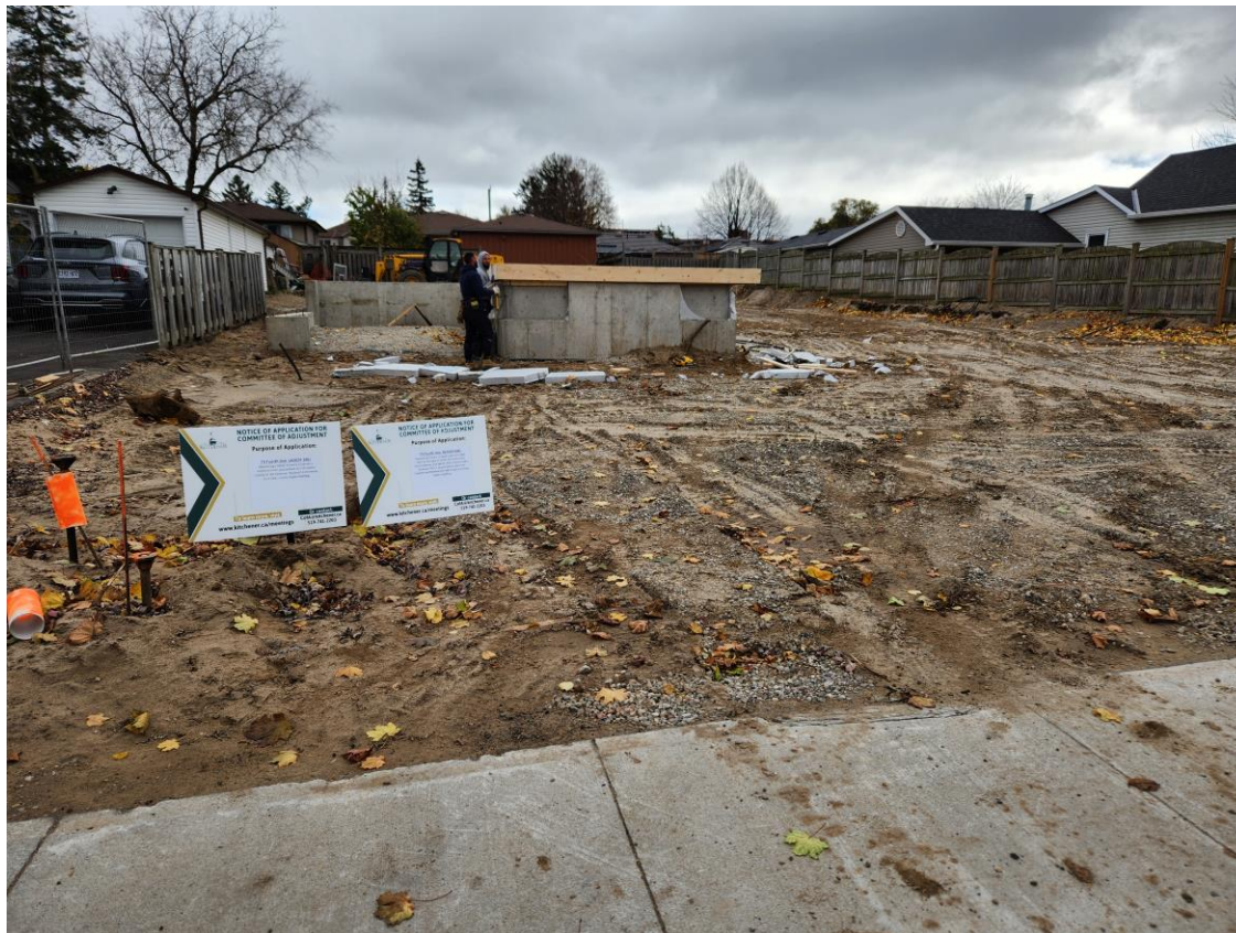
Figure 4: Subject Property and Foundation for Single Detached Dwelling on Retained Lot
