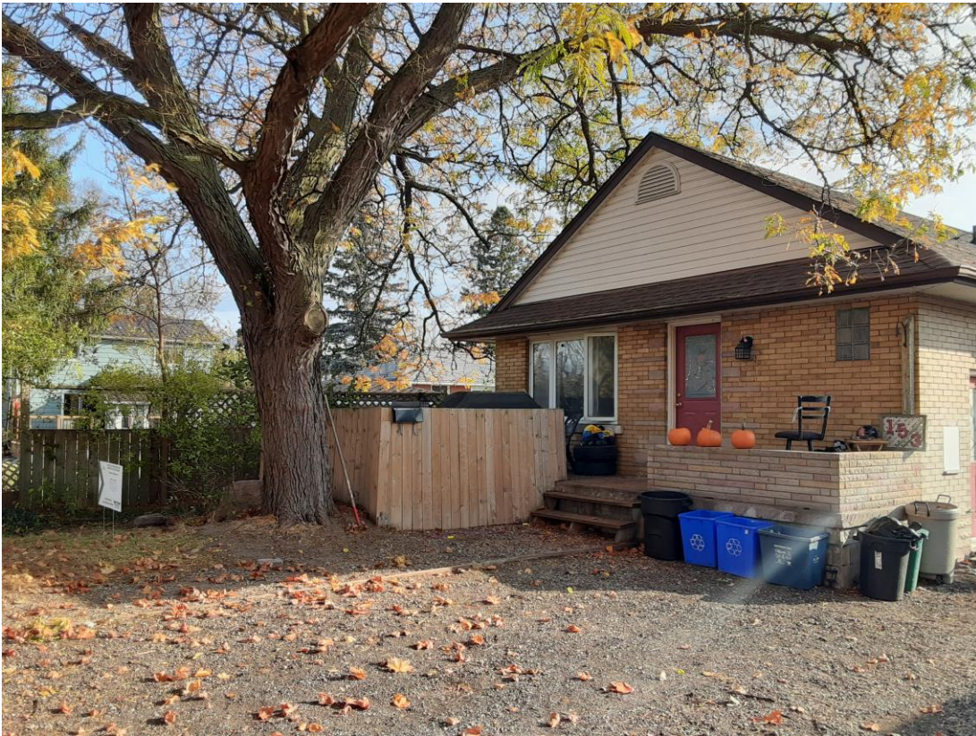
Figure 6 - Existing front yard fence. Height 1.5 metres (4 ft, 11 in).
