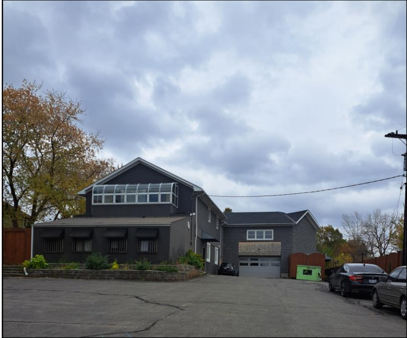
Figure 4: Front of the Existing Building
