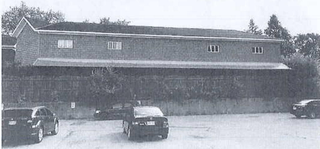
165 Fairway Road North (Side View)
