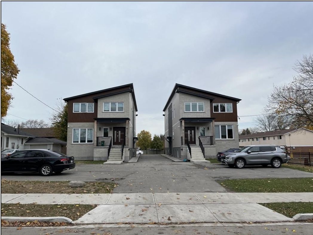
Figure 2: View of Subject Lands from Rutherford Drive (November 5, 2024) (70 Rutherford Drive- left side, 74 Rutherford Drive- right side)
