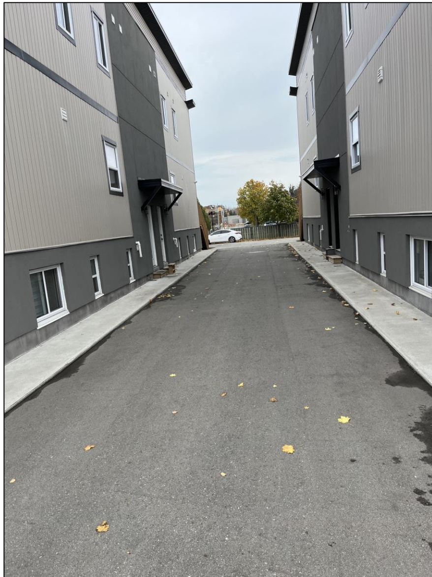
Figure 3: View of existing Shared Driveway access to rear (November 5, 2024)
