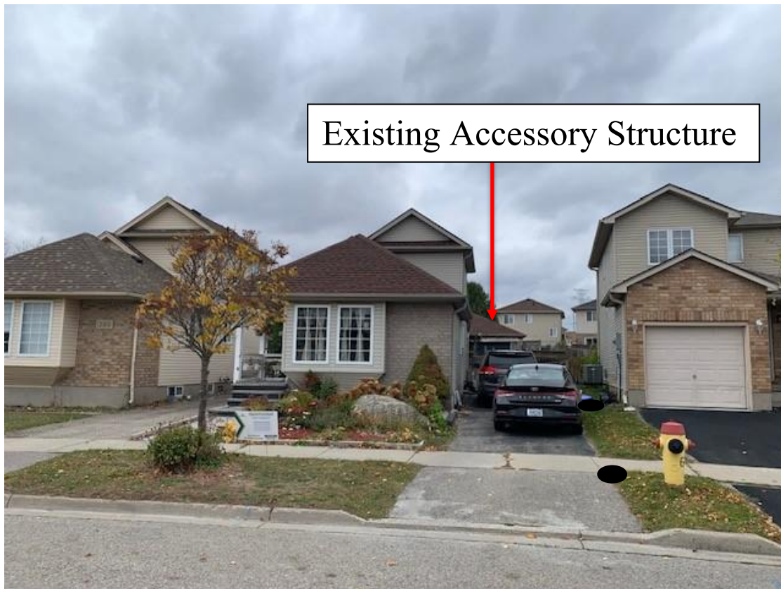
Figure 8: Existing Site Conditions at 386 Wake Robin Crescent on October 31, 2024.
