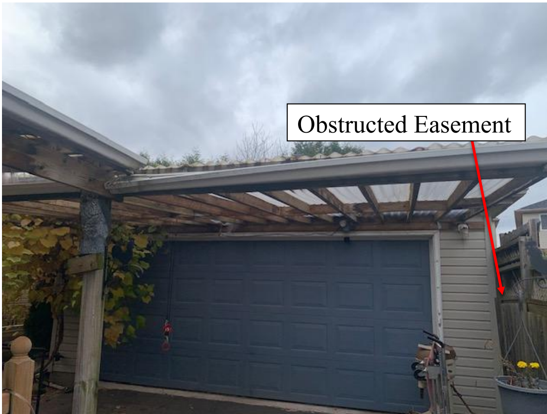
Figure 9: Existing Accessory Structure at 386 Wake Robin Crescent on October 31, 2024.
