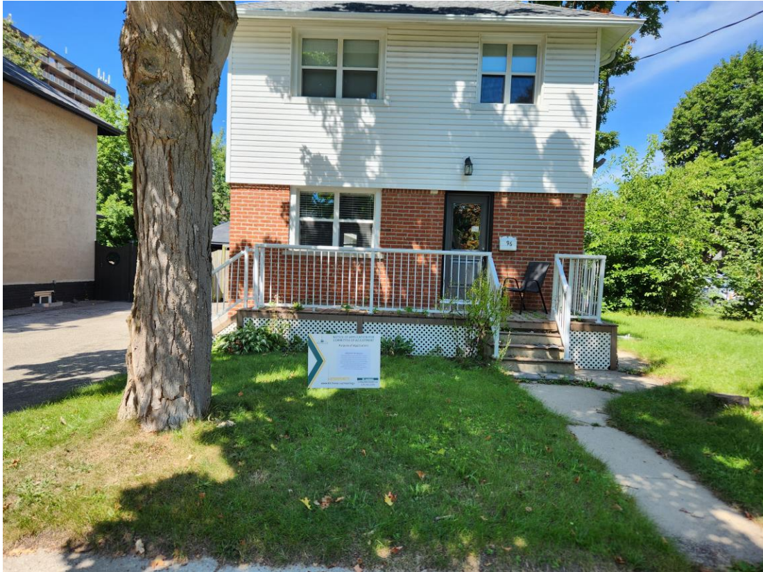
Figure 4: Front of Existing House (Wood Street Façade)
