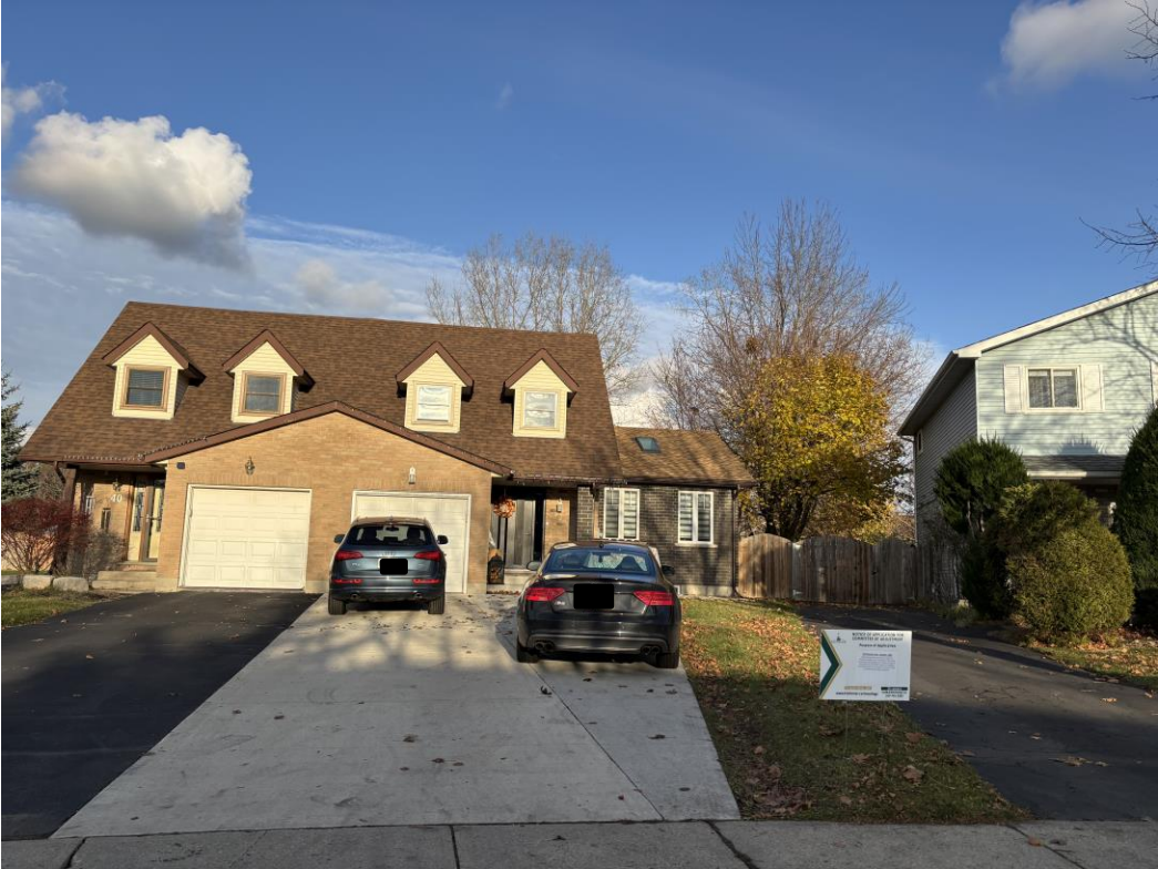
Figure 4 – View of 42 Wendy Crescent from the street.
