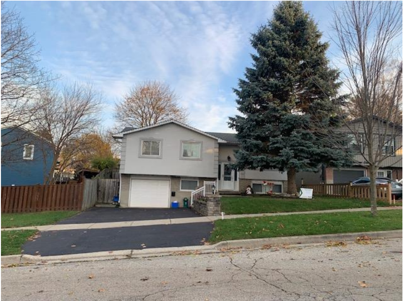
Figure 3 – View of 25 Sandsprings Crescent from the street.
