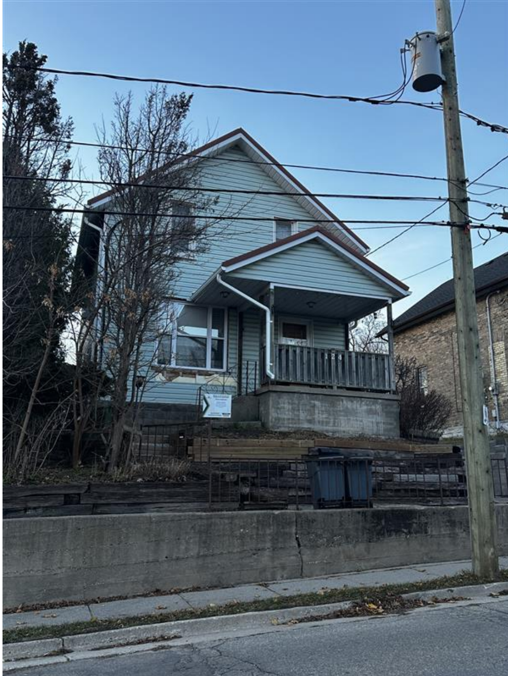
Figure 5: Existing Site Conditions - 124 Cedar Street South on November 18, 2024
