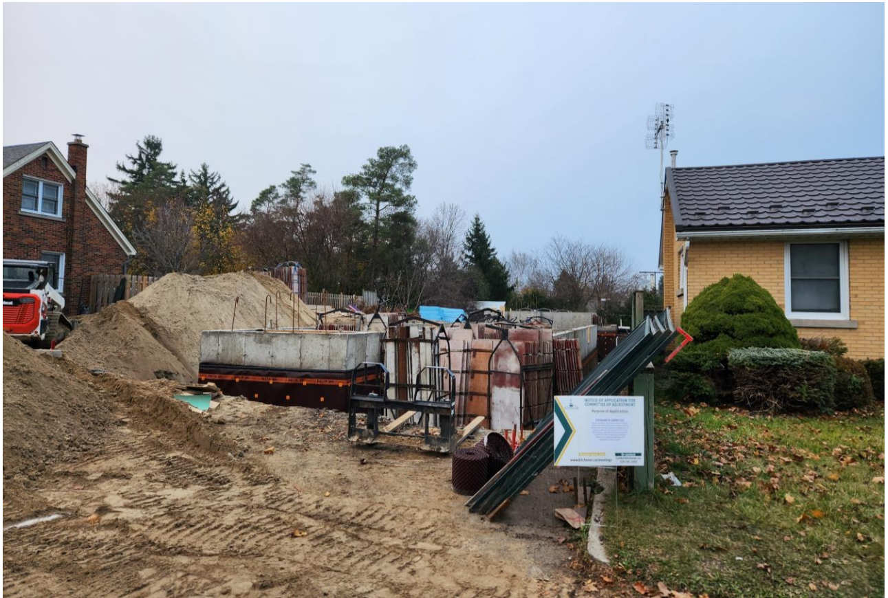
Figure 4: Proposed Single Detached Dwelling Under Construction
