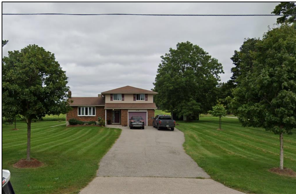
Figure 4: The Existing Dwelling Street View
