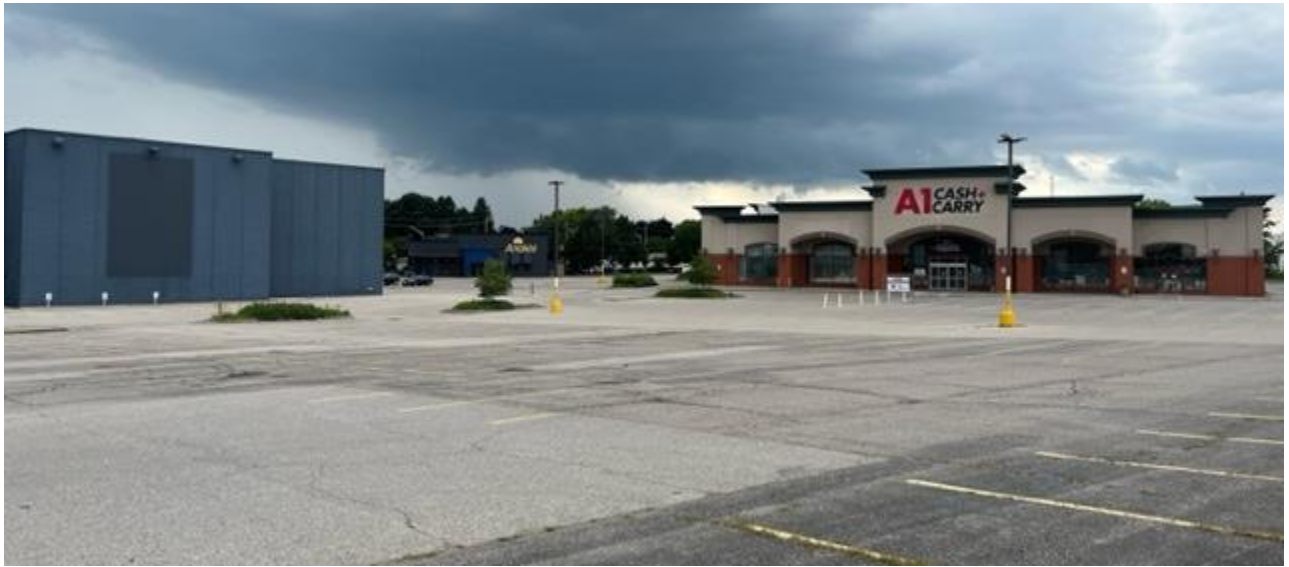
Figure 6: Existing building and existing conditions
