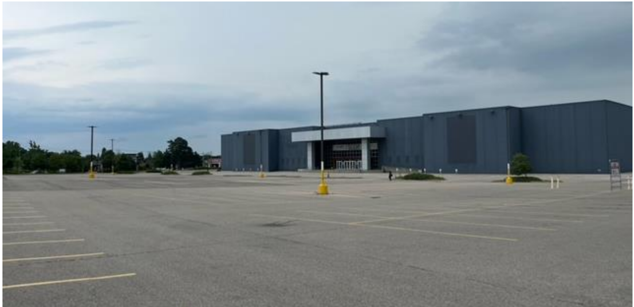
Figure 7: Existing building and existing conditions
