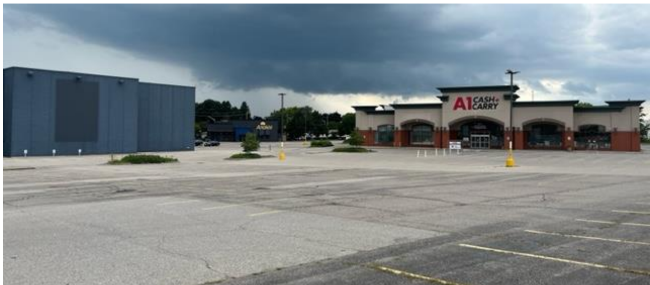
Figure 4: Existing building and existing conditions
