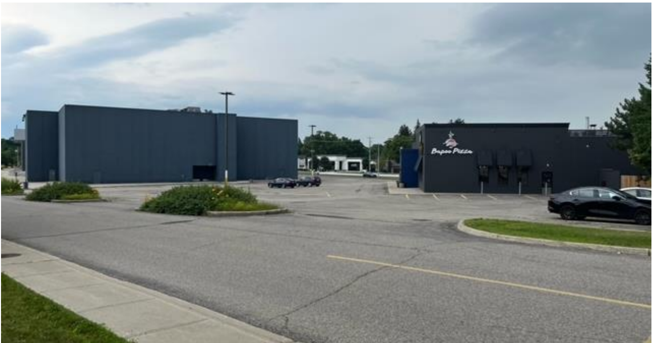
Figure 6: Existing buildings and existing conditions
