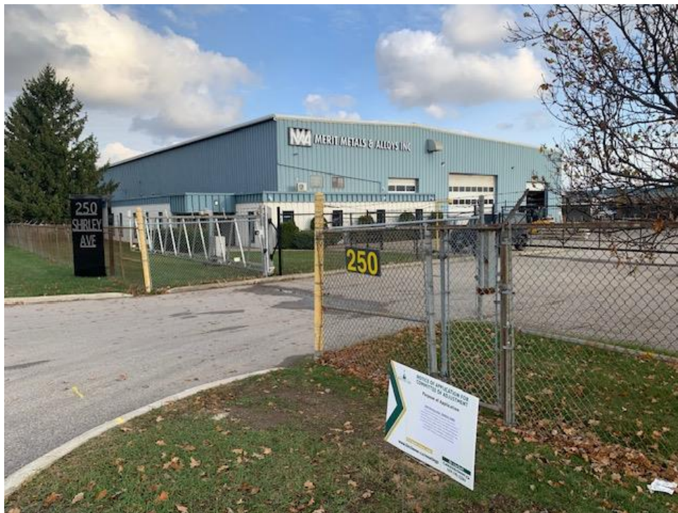
Figure 3: Existing Industrial Facility at 250 Shirley Avenue on November 21, 2024
