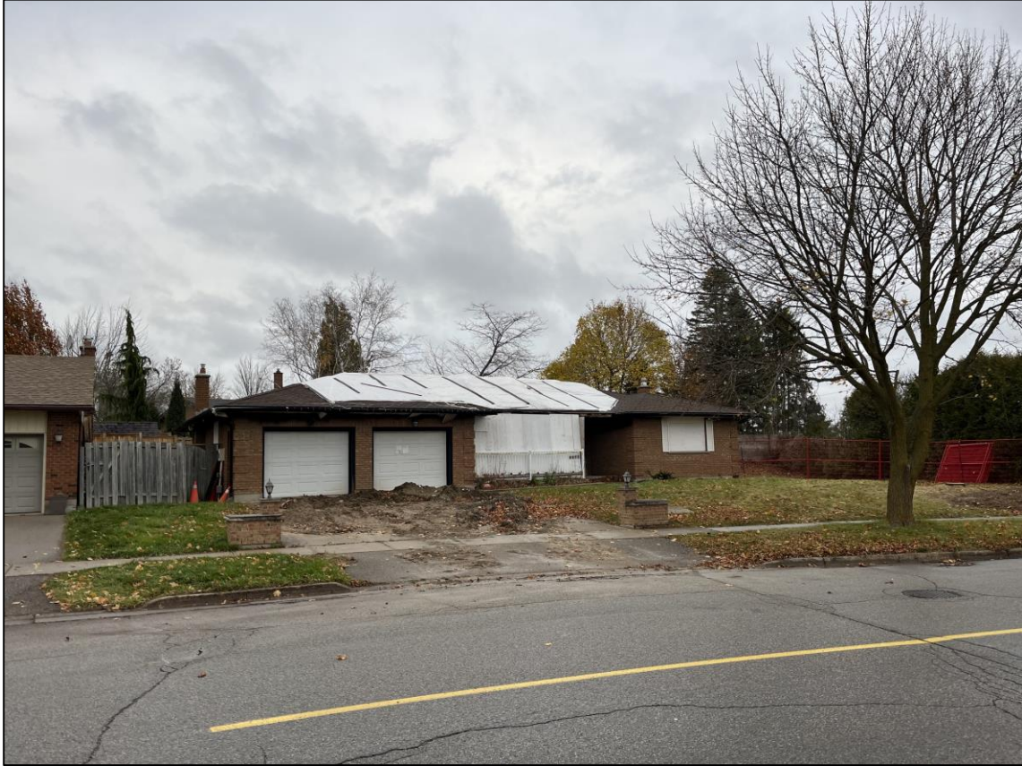
Figure 2: View of Single Detached Dwelling with Fire Damage (March 27, 2024)
