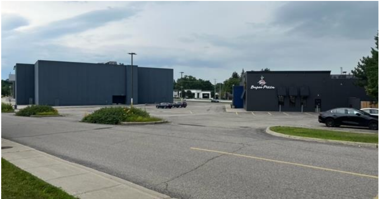
Figure 8: Existing buildings and existing conditions
