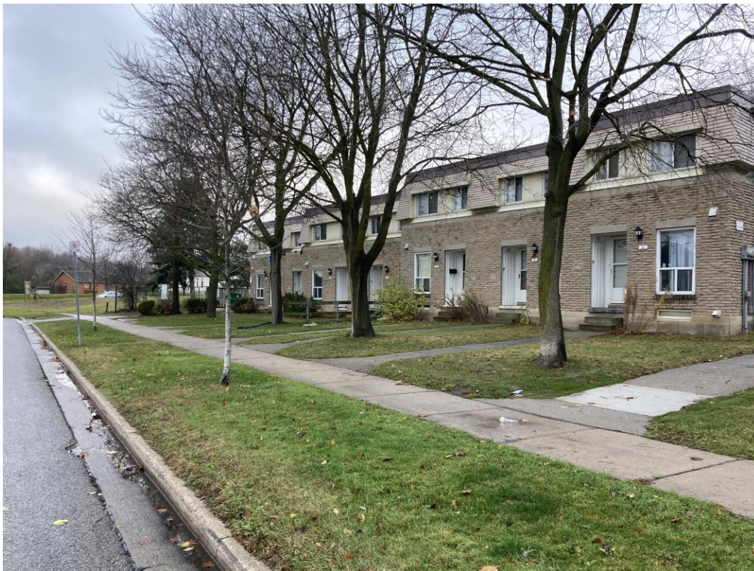
Figure 6: Existing Site Conditions at 15-105 Mooregate Crescent on November 26, 2024.
