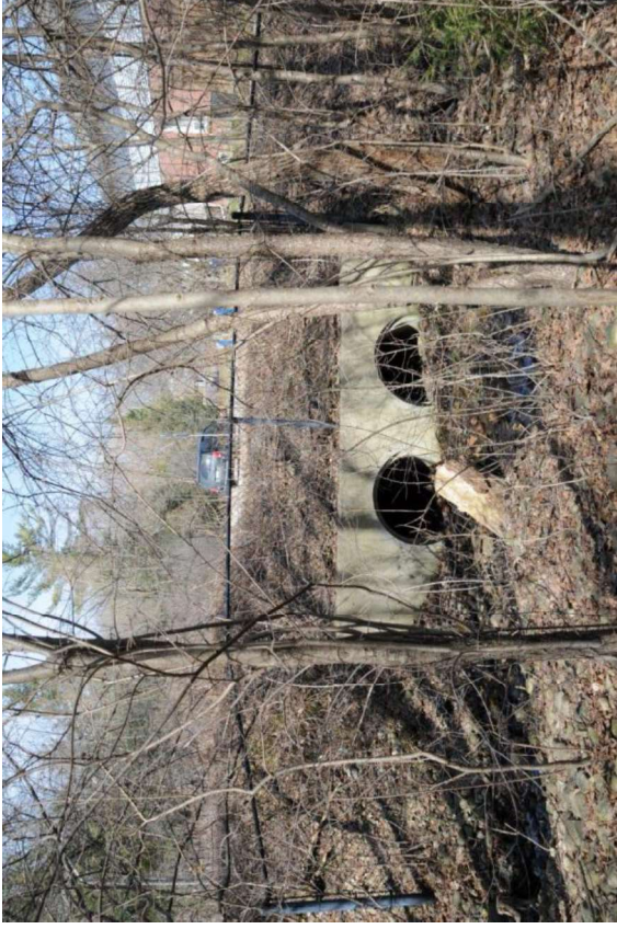
Twin 1.2 m culverts (above) with a river stone entrance apron at the headwall (below) cross under the Biehn Drive cul-de-sac and connect to a permanent Strasburg Creek tributary to the north
