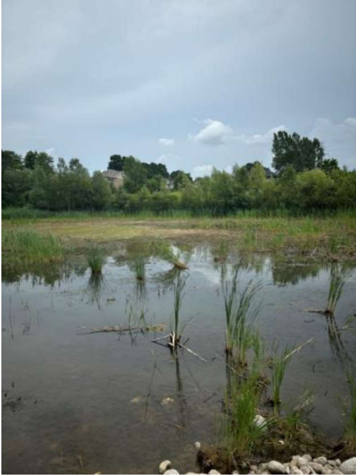
Photo 5: Hearthwood Stormwater Wetland - Main Embayment Looking Northwest
