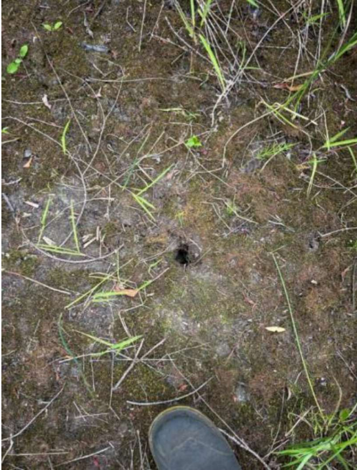
Photo 9: Hearthwood SWM Infiltration Trench - Gabion Stone can be seen Through Hole
