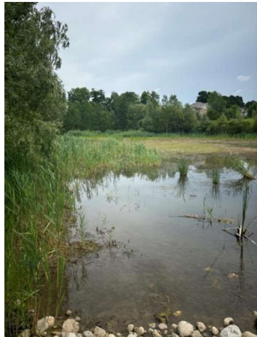
Photo 4: Hearthwood Stormwater Wetland - Main Embayment Looking West from Outlet
