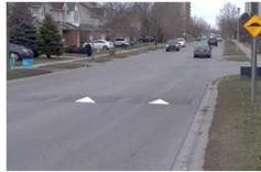
Speed Humps/Cushions or Raised Crosswalks
