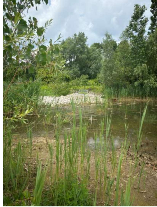
Photo 2: Hearthwood Stormwater Wetland - Outlet Point
