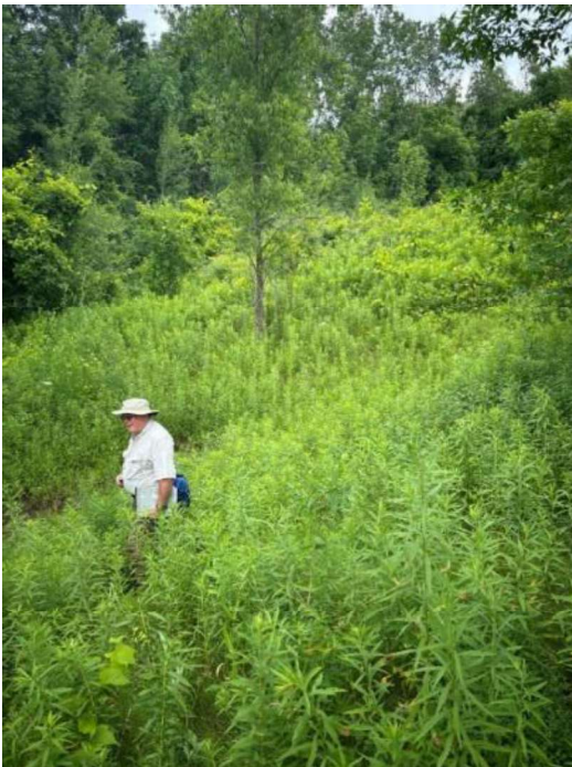
Photo 11: Fill Slope Mounded Up Outside of SWM Pond
