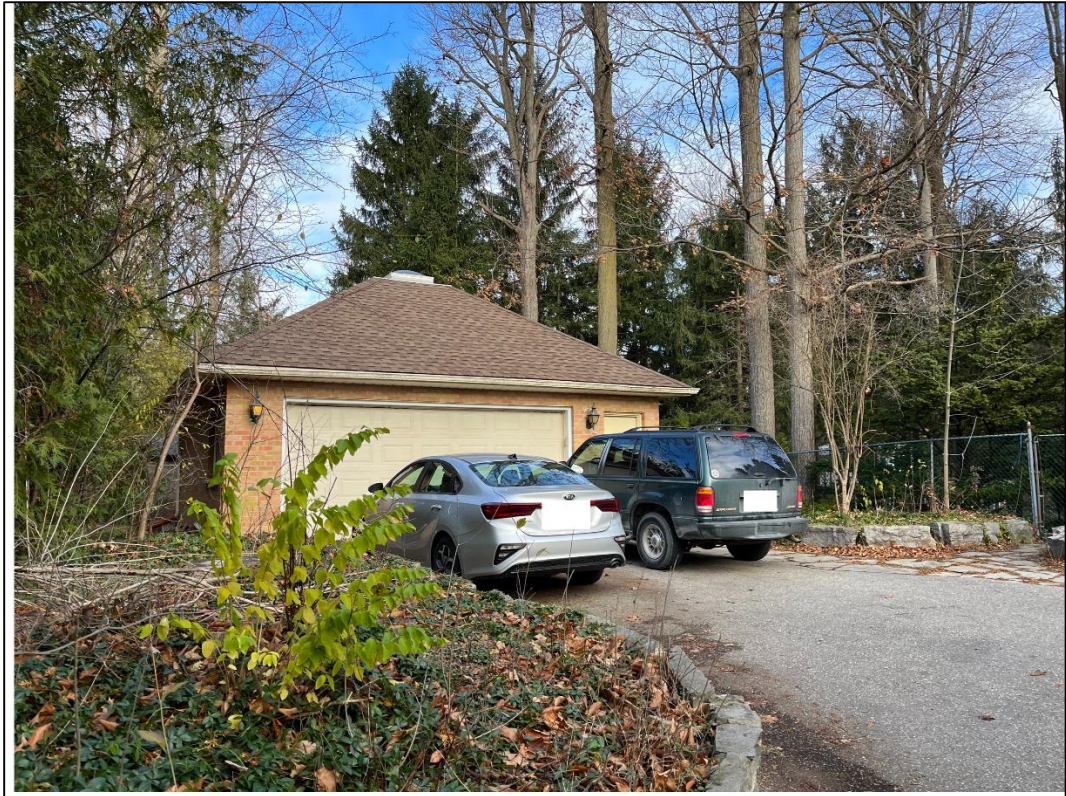
Figure 4: View of Existing Detached Garage
