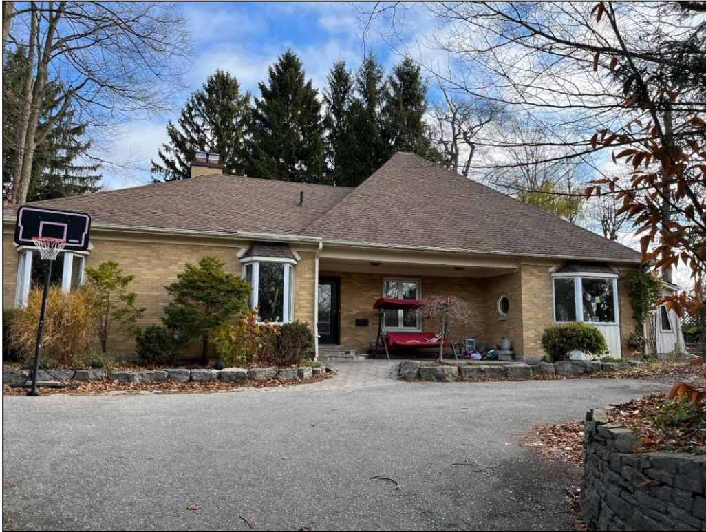
Figure 3: View of Existing Single Detached Dwelling
