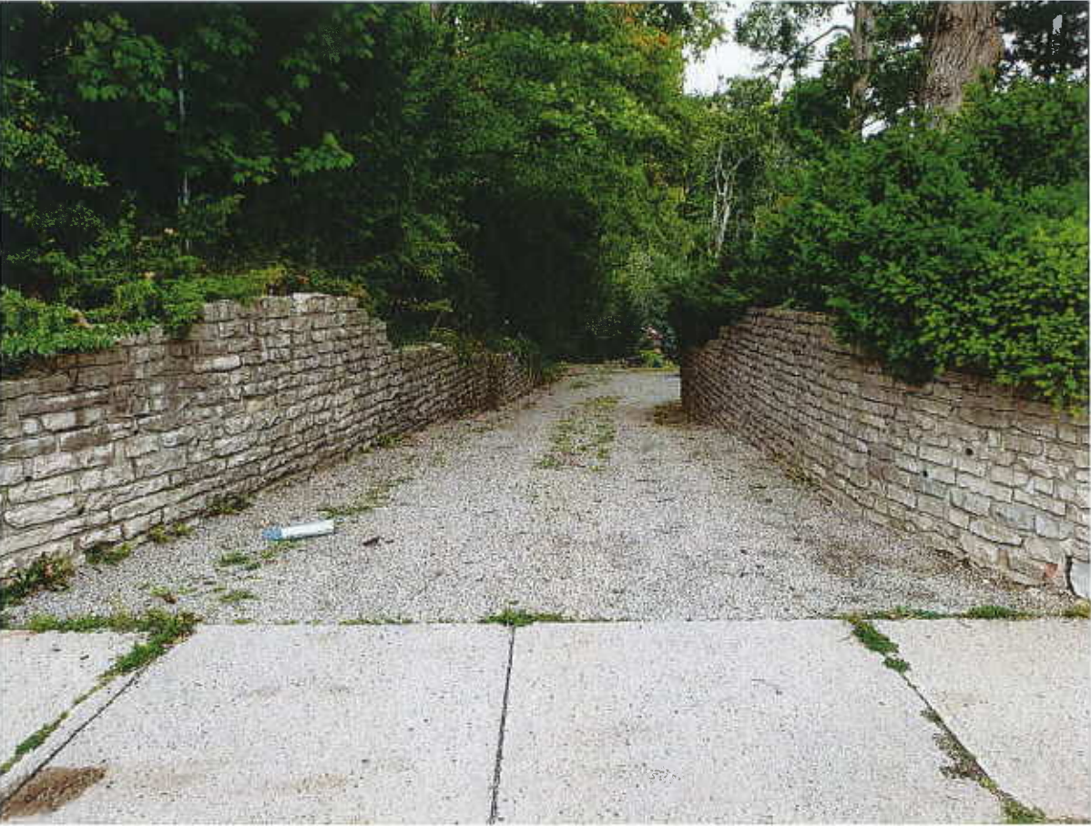
View looking down driveway into the property from Westwood sidewalk with chain-link fence post (property line) visibly embedded in common boundary area
