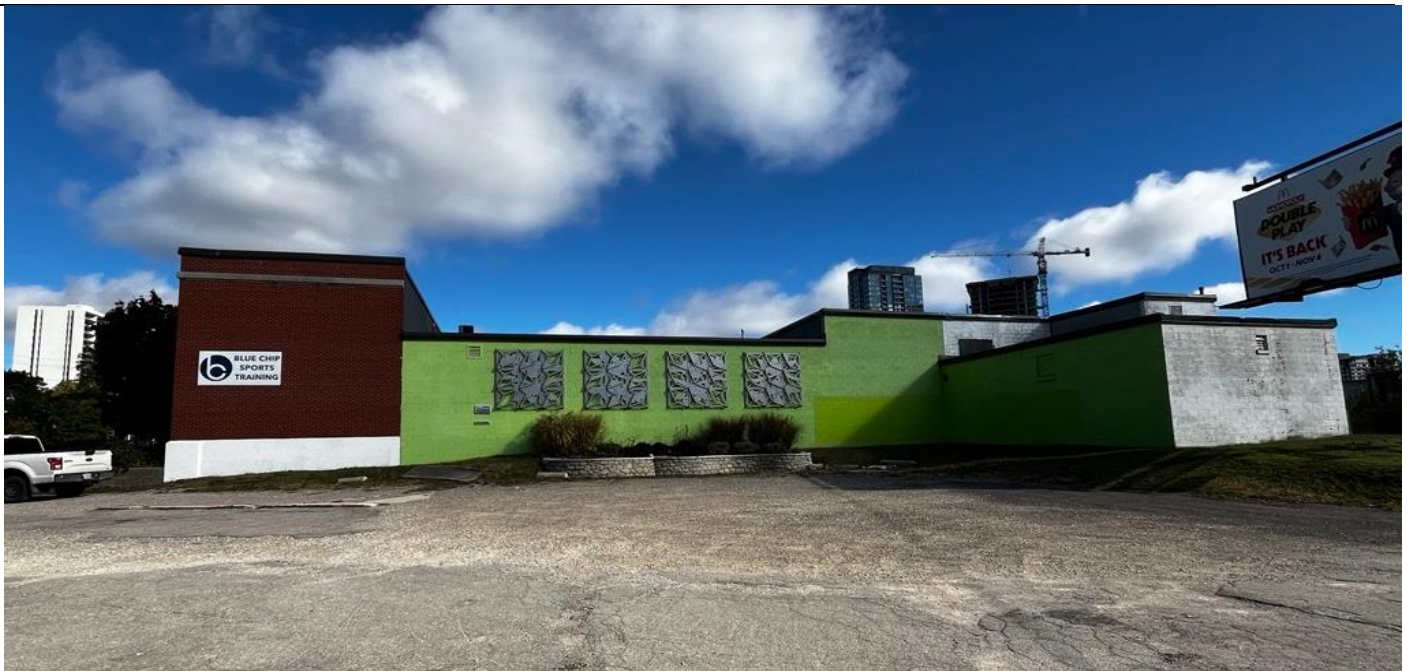
South-Side Façade (1927 Portion and new addition)
