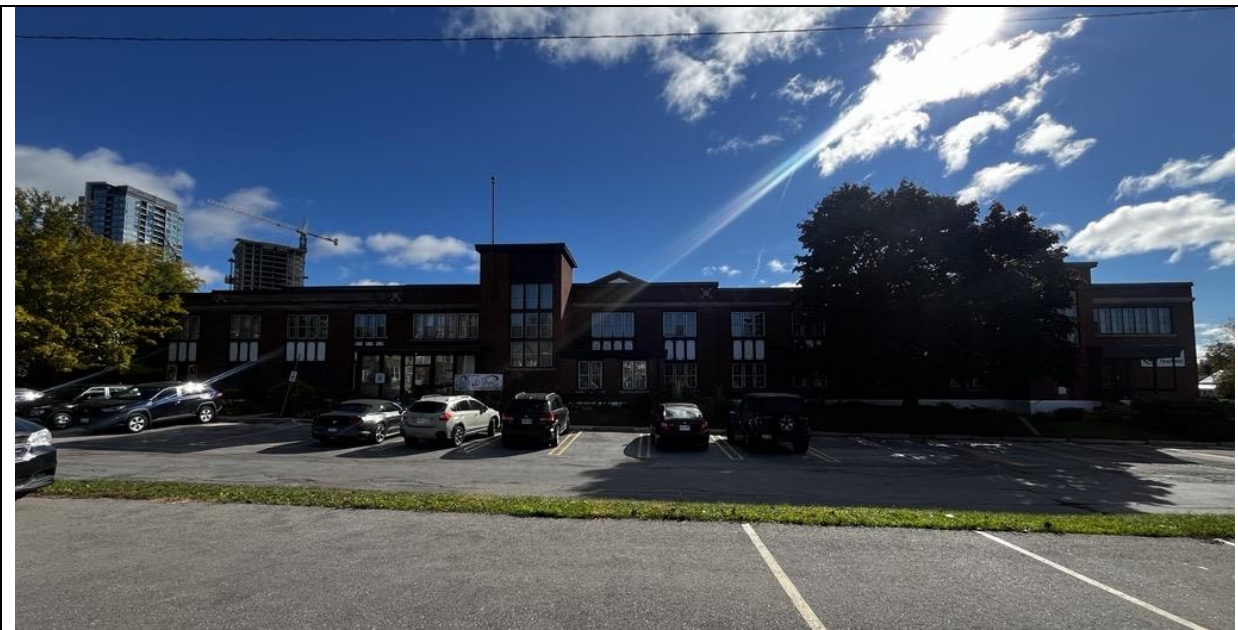
Front Façade of Subject Building
