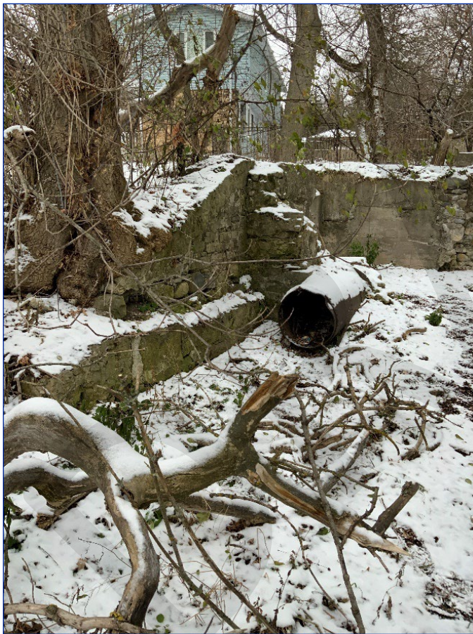
Photo 47: Channel sidewall return corner with metal pipe
