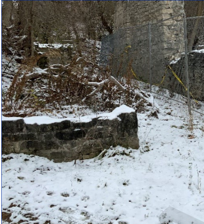
Photo 48: Small foundation section at east end
