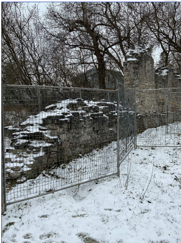
Photo 38: Remaining wall; east end of south elevation
