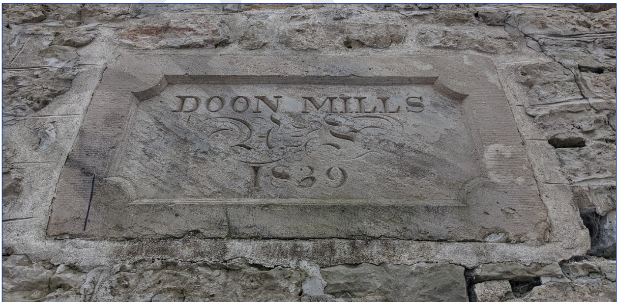
Photo 23: View of the date stone near the top of the western end of the south elevation
