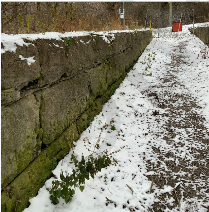
Photo 46: Mill race east sidewall (typical)
