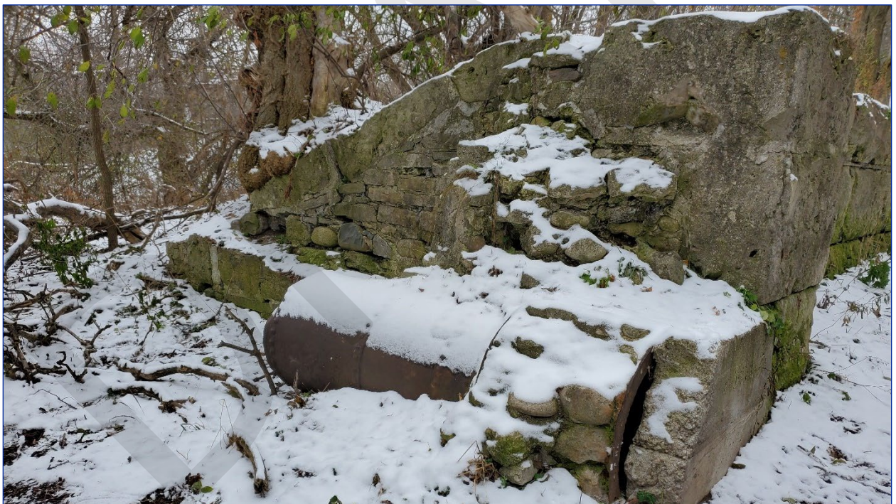
Photo 27: View southeast of the mill race and metal tube
