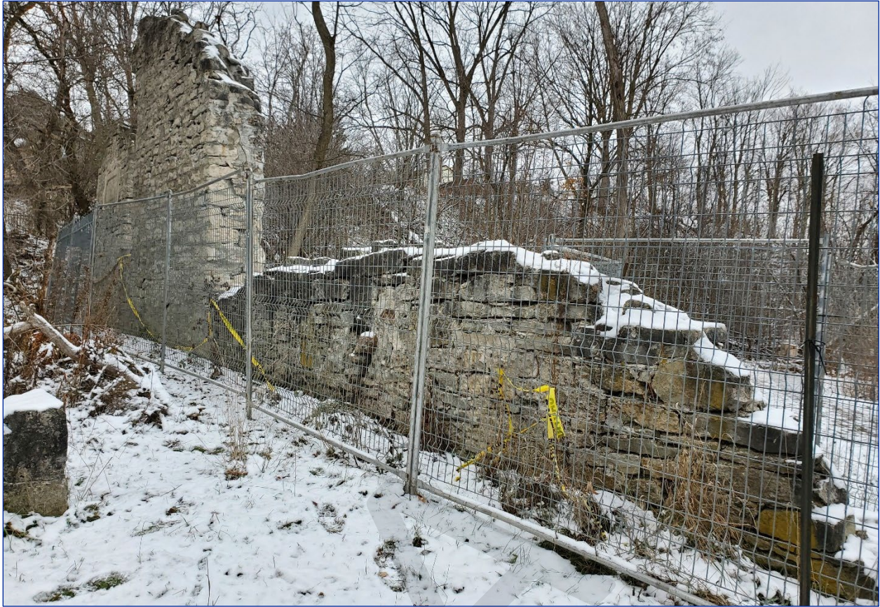
Photo 22: View of the south elevation of the mill ruins
