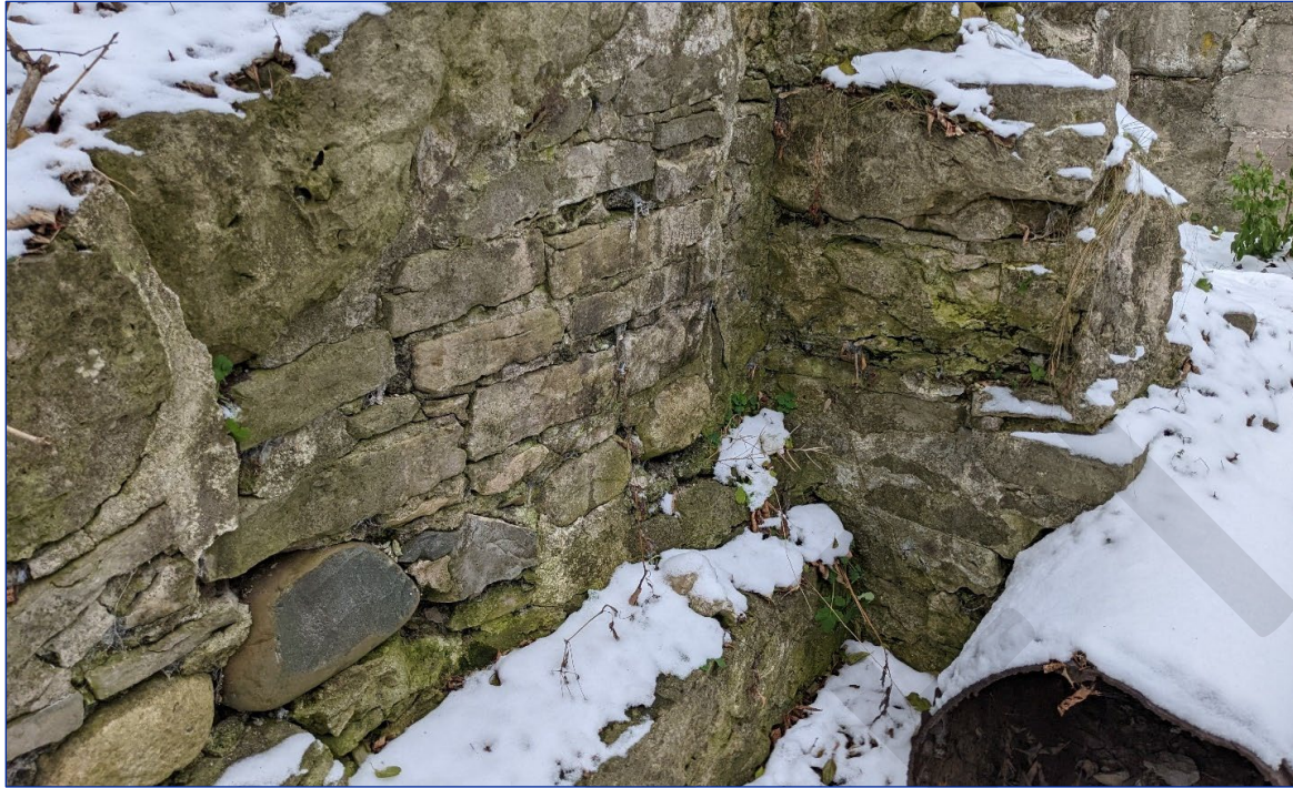
Photo 28: View southwest of the mill race and metal tube
