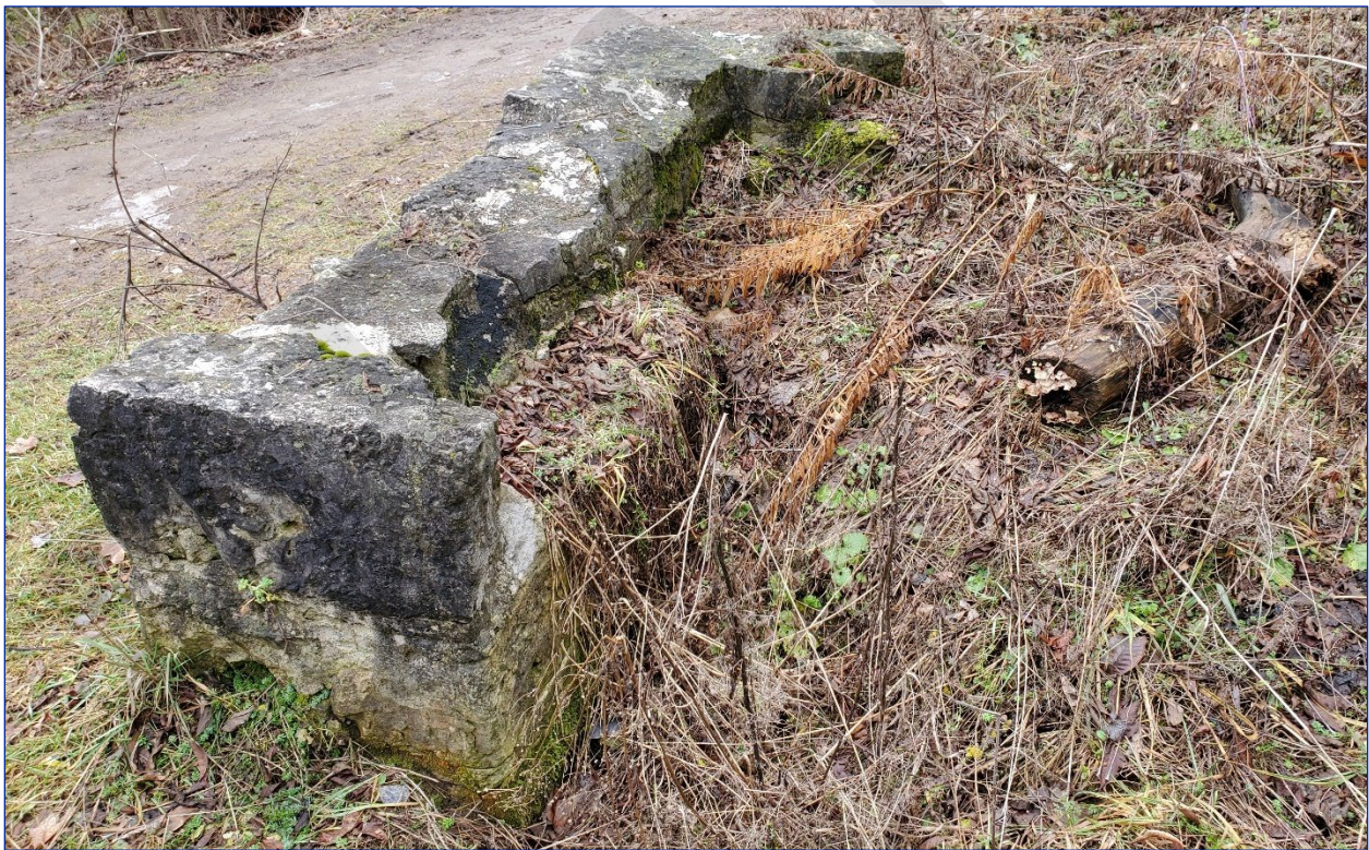
Photo 33: View southeast of the partial wall and foundation
