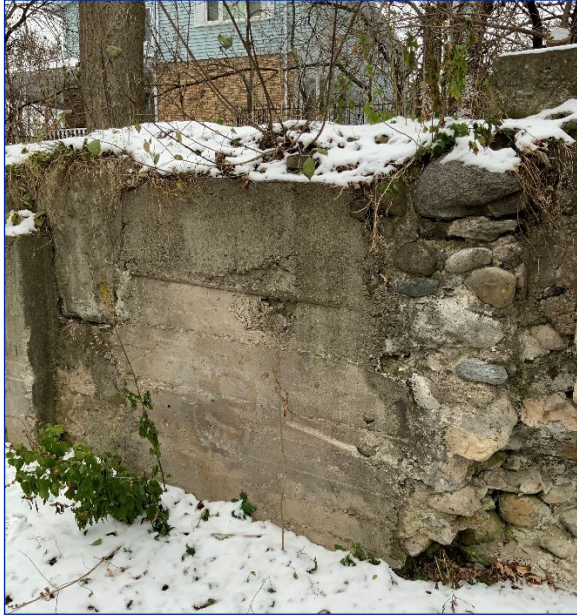
Photo 45: Cast-in-place concrete, west mill race sidewall
