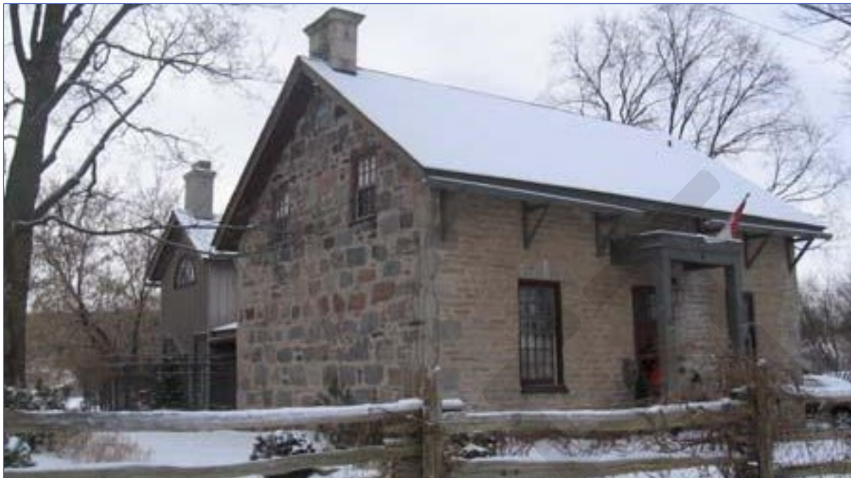
Photo 6: Northeast view of 39 Doon Valley Drive 93
