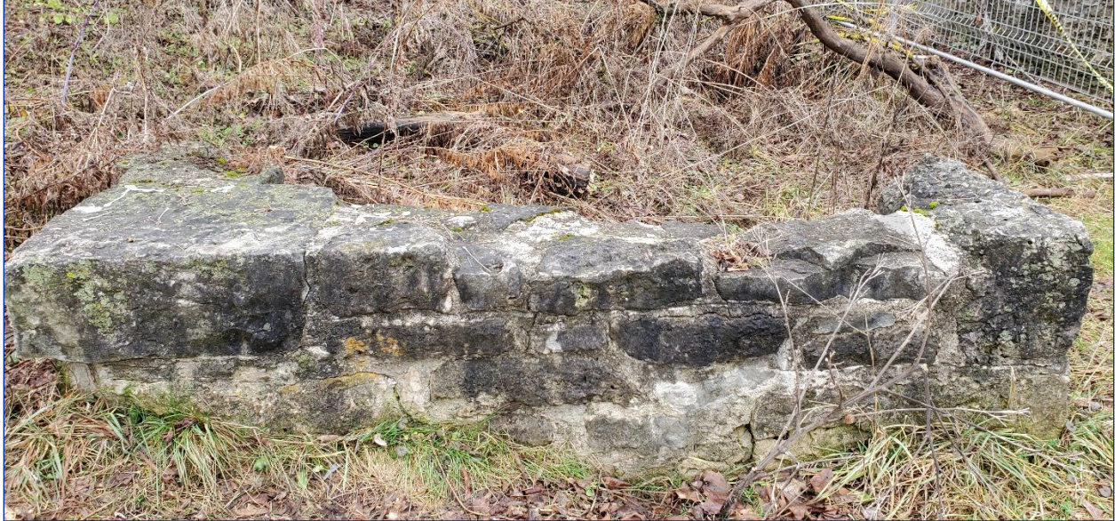
Photo 32: View west of the partial wall and foundation
