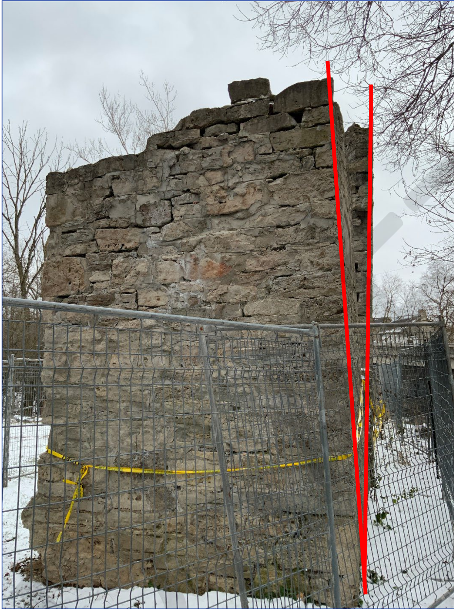
Photo 42: View along south elevation; taken from west corner looking east
