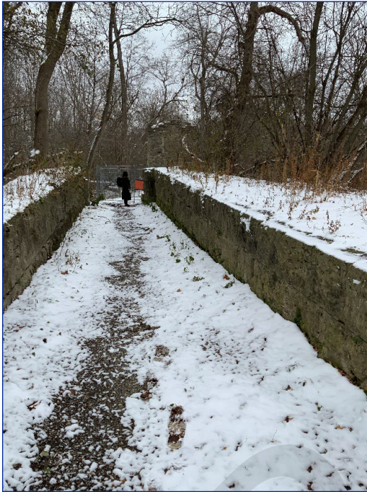
Photo 44: A channel—possibly a Mill race—looking north
