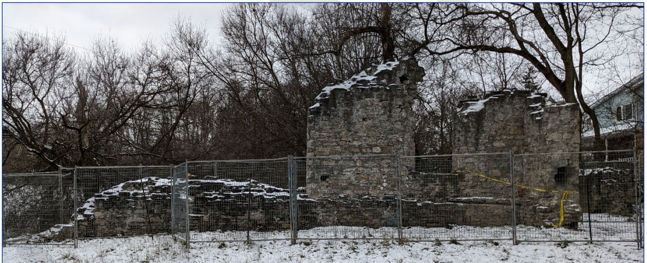
Photo 21: View of the north elevation of the mill ruins (formerly the interior)
