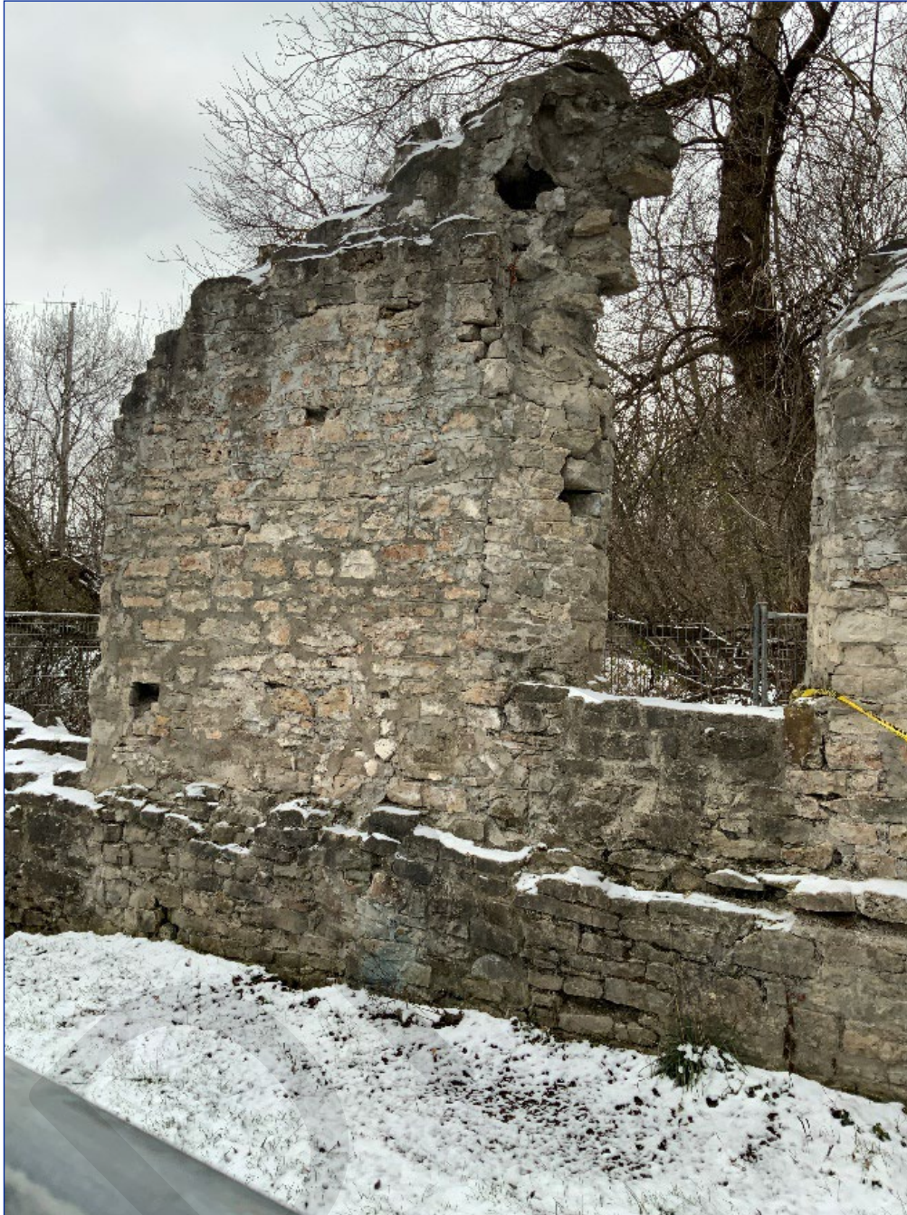
Photo 41: Free standing section of wall; south elevation
