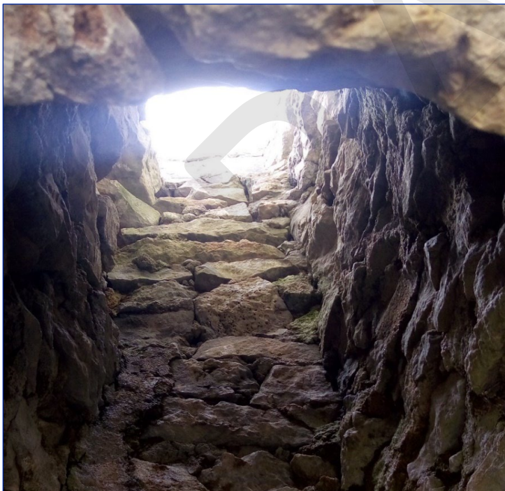
Photo 25: View up the shaft in the west elevation wall in 2019 123
