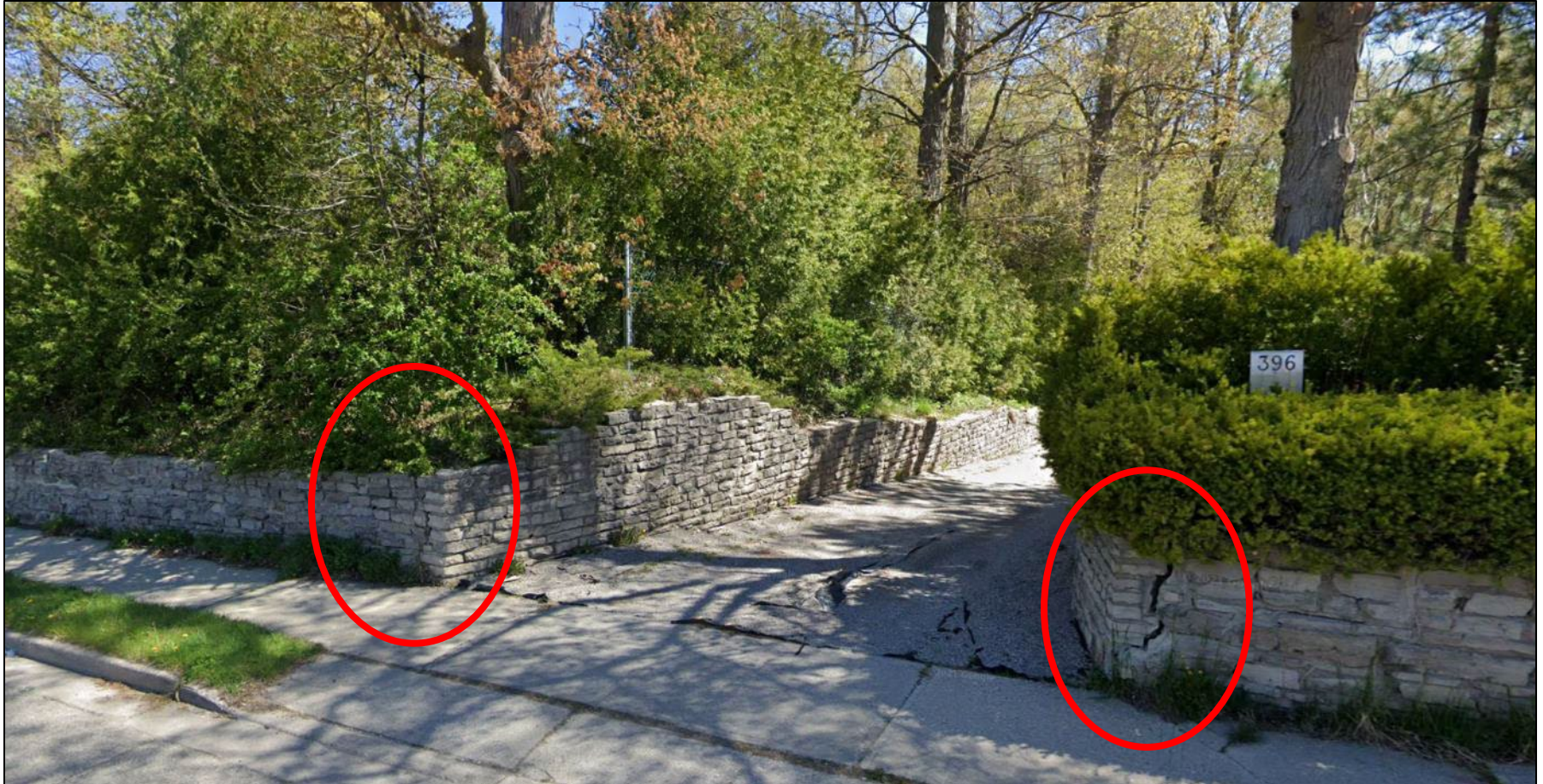
Source: Google Streetview – May 2021
