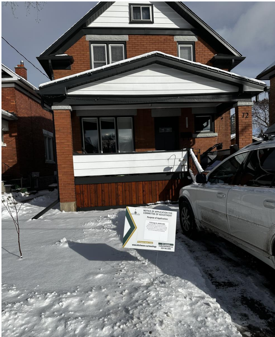
Figure 7: Existing Site Conditions as of January 3, 2025
