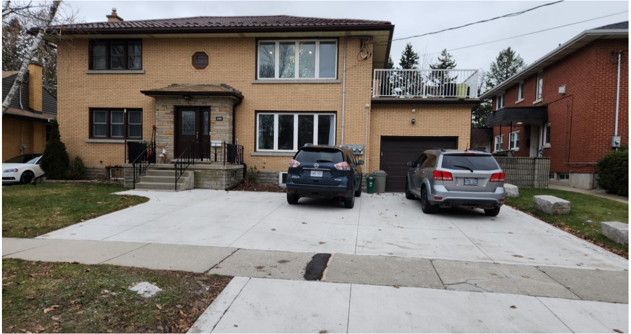
Figure 4: 240 Chapel Street (Edge of Driveway on Both Sides Proposed as Walkway)
