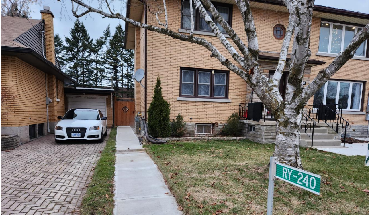
Figure 5: Walkway Leading to Existing and Proposed Additional Dwelling Unit
