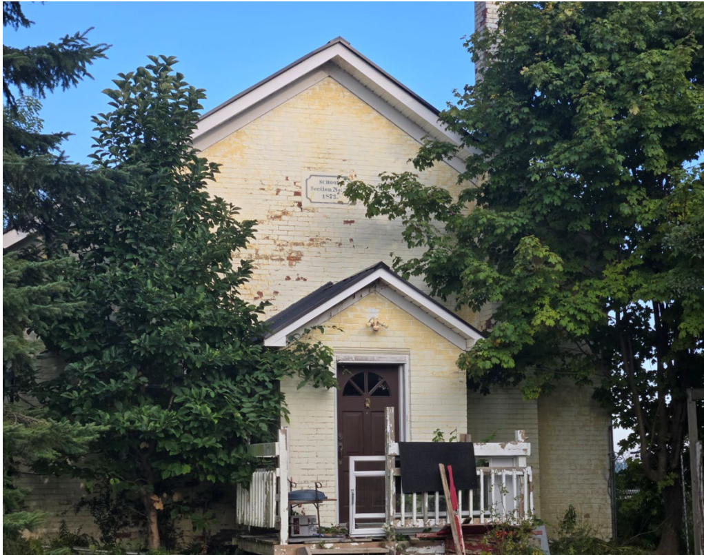
Figure 7: View of the structure on the listed property located at 1970 Fischer-Hallman Road. (MHBC, 2024)
