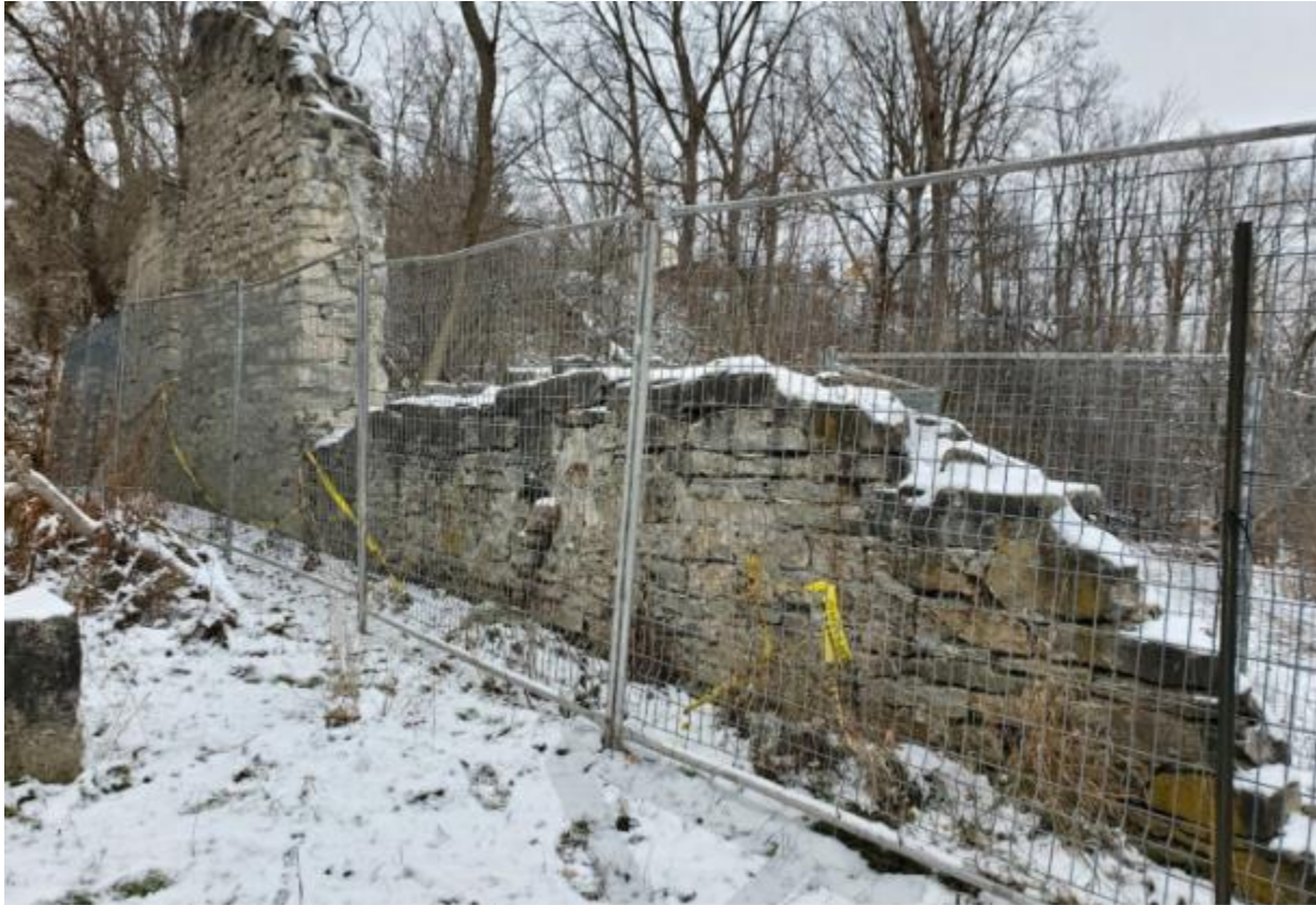
Figure 3. View of the south elevation of the ruins. (Source: Lower Doon Mill Ruins CHER)
