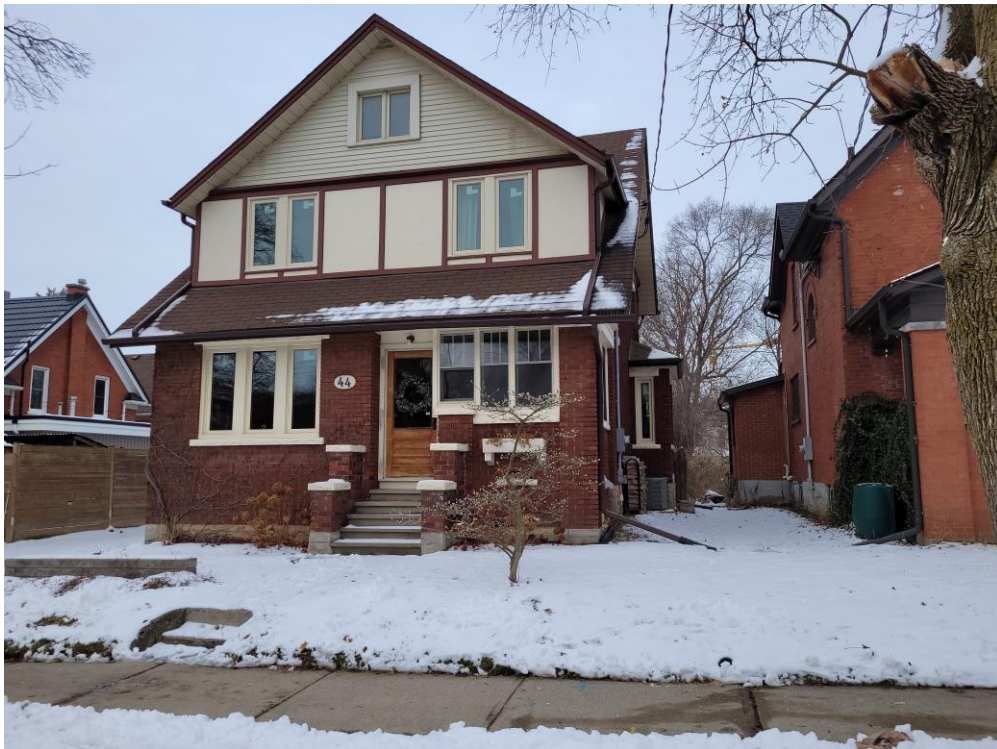
Figure 4 - Photo of 44 Betzner Avenue North
