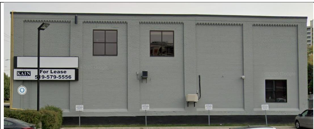
Side Elevation (West Façade): 241-247 Duke Street West / 55 Victoria Street North (Google, 2024)
