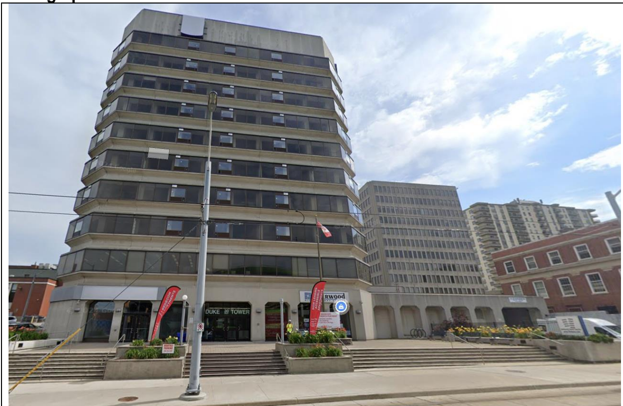
Front Elevation (South Façade) (Google, 2024)
