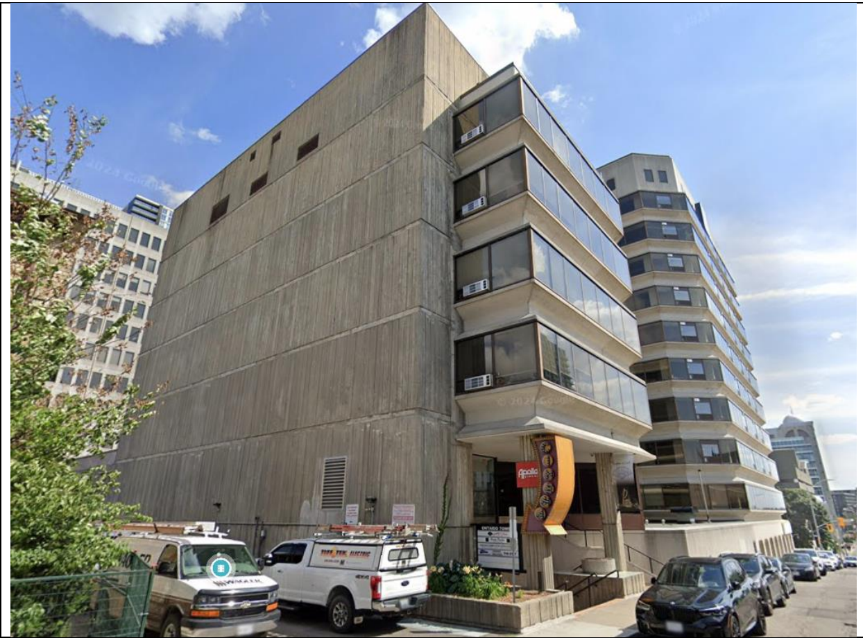
Rear Elevation (North Façade) (Google, 2024)
