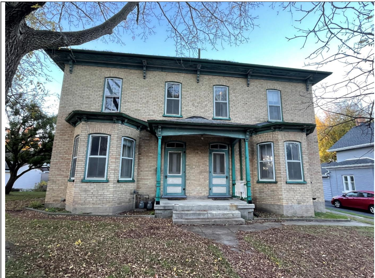
Front Elevation (North Façade) – 79-81 St. George Street
