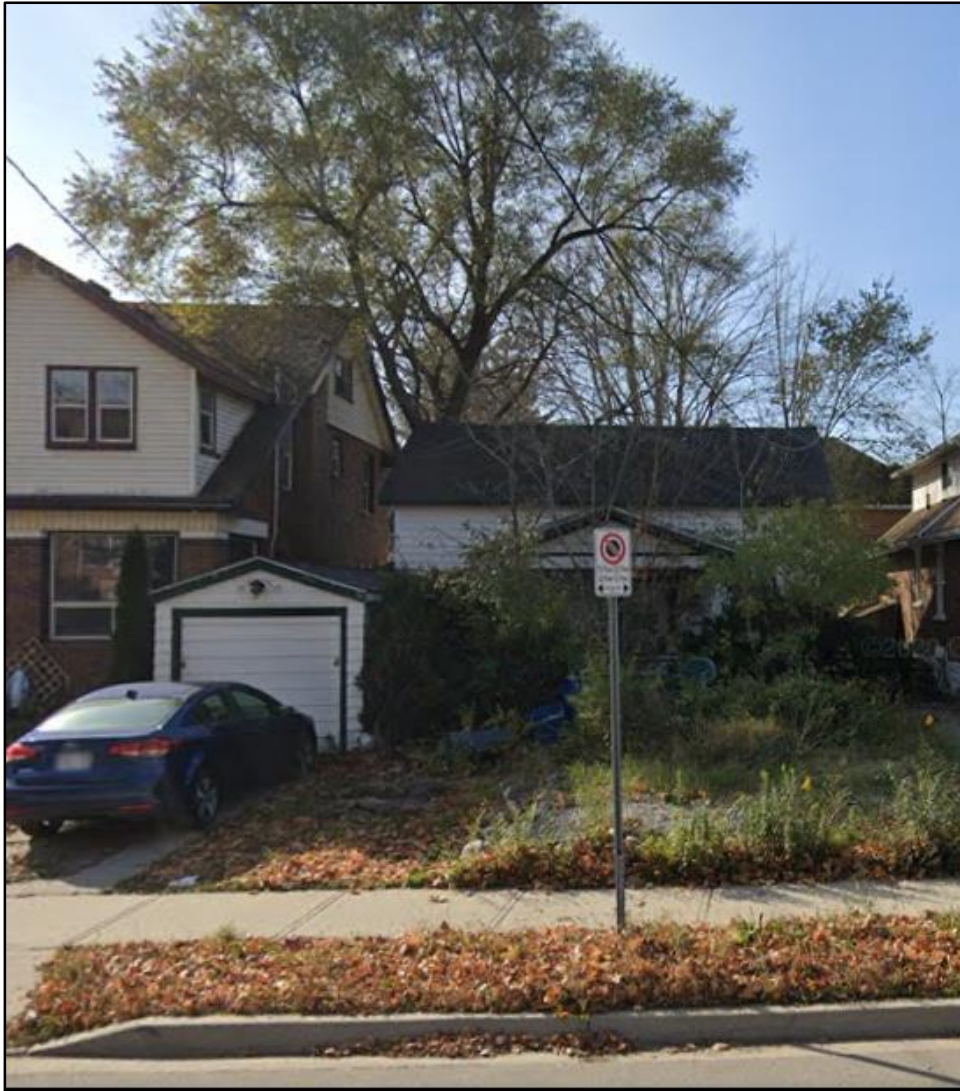
Photo 1: Exterior Facing Courtland Ave
