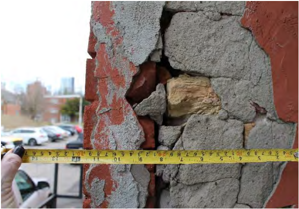
Figures 40 & 41: (left) View of poor masonry repairs at exterior of building 1, (right) View of deteriorated/spalled masonry at exterior of Building 1 (MHBC, 2024)
