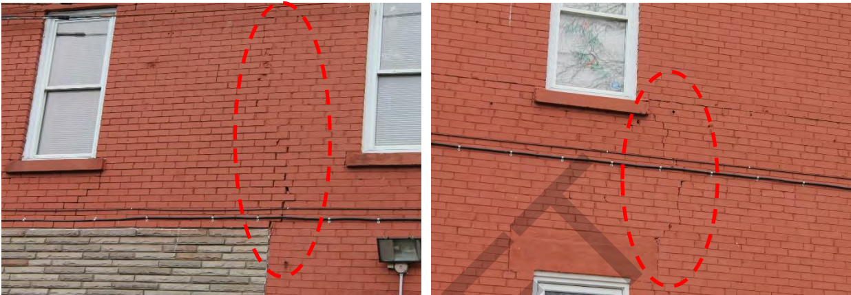
Figures 36 & 37: Photos of settlement cracks at the exterior of Building 1, (MHBC, 2024)
