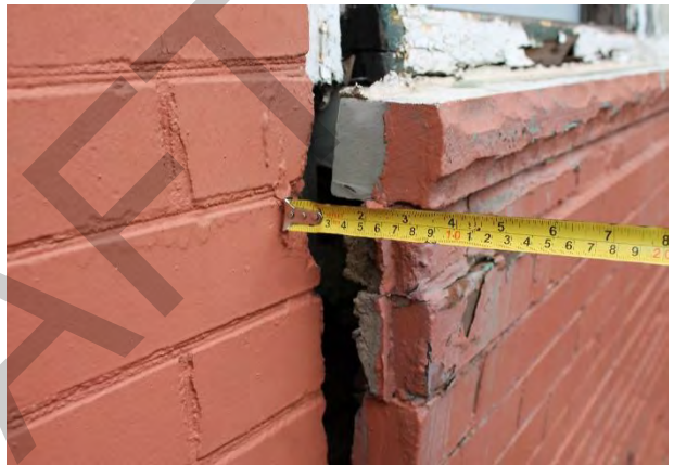
Figures 42 & 43: (left) Secondary view of broken and deteriorated masonry at exterior of Building 1, (right) View of cracks in masonry wall at exterior of Building 2, (MHBC, 2024)
