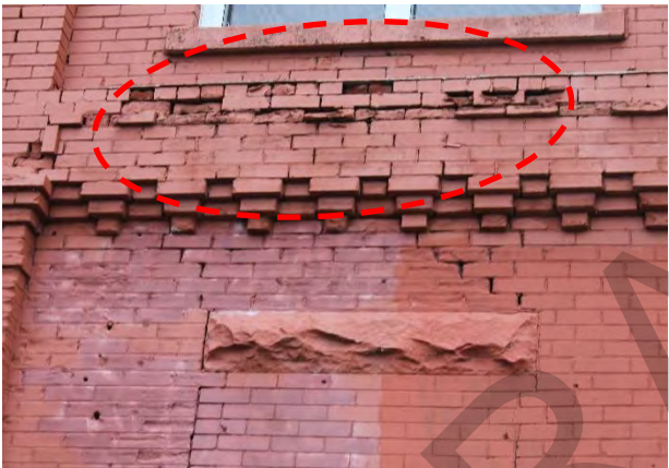
Figures 42 & 43: (left) Secondary view of broken and deteriorated masonry at exterior of Building 1, (right) View of cracks in masonry wall at exterior of Building 2, (MHBC, 2024)
