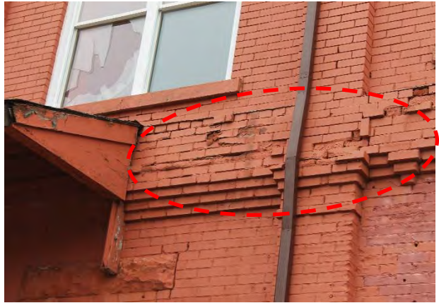
Figures 40 & 41: (left) View of poor masonry repairs at exterior of building 1, (right) View of deteriorated/spalled masonry at exterior of Building 1 (MHBC, 2024)
